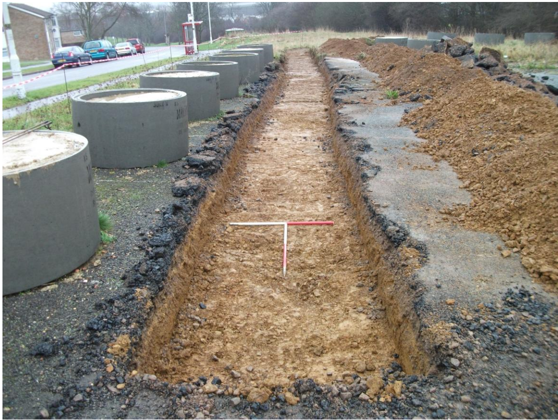
Trench 3, looking north-east
