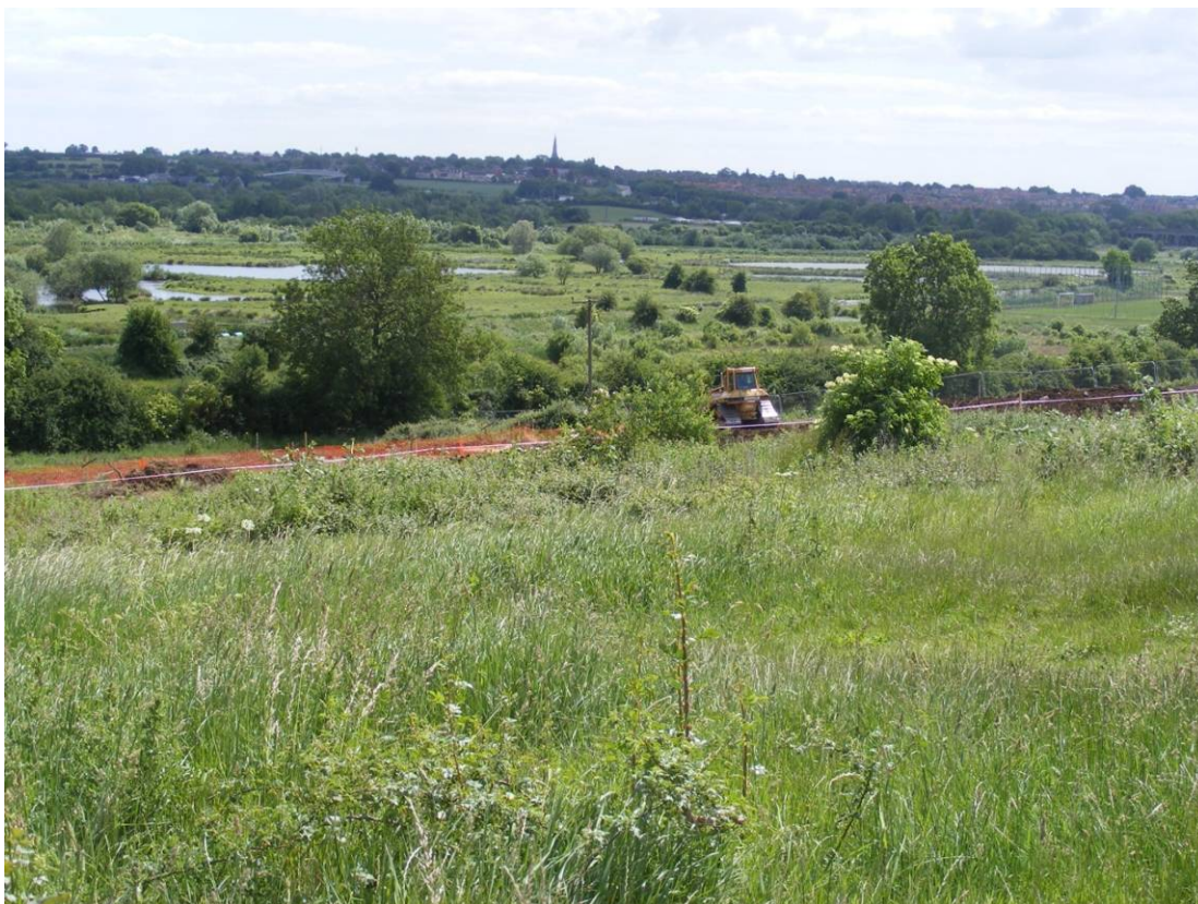
Plate 1: General view of the site during groundworks
