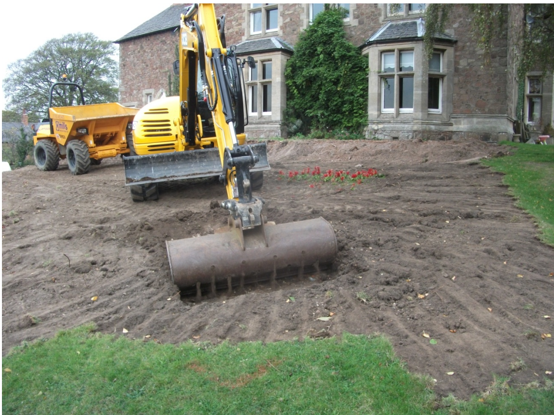
The groundworks in progress, looking north Fig 5
