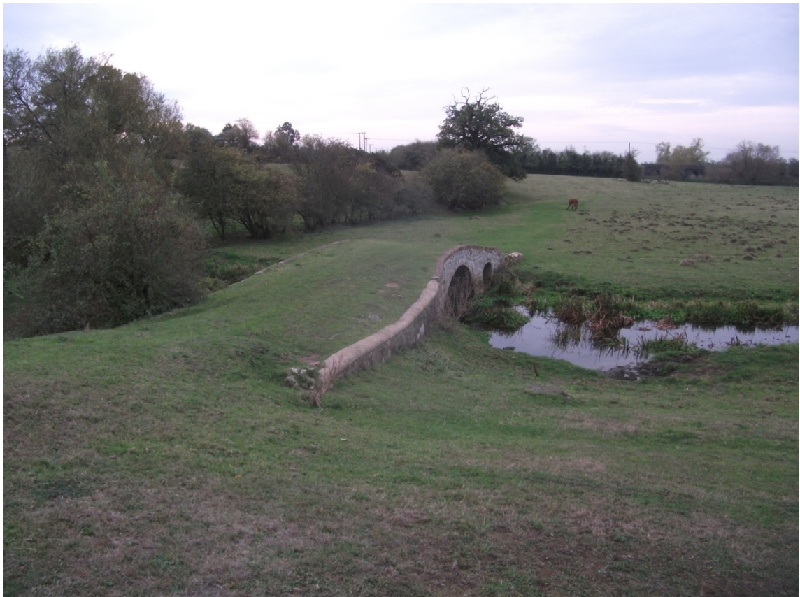
The bridge crossing the River Soar, looking south Fig 4
