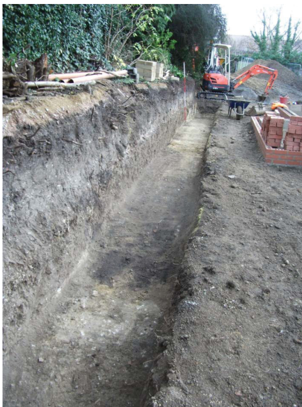
The retaining wall foundation trench Fig 5
