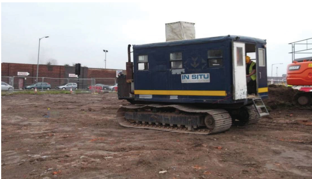
Site investigation bomb survey by IN SITU, looking south
