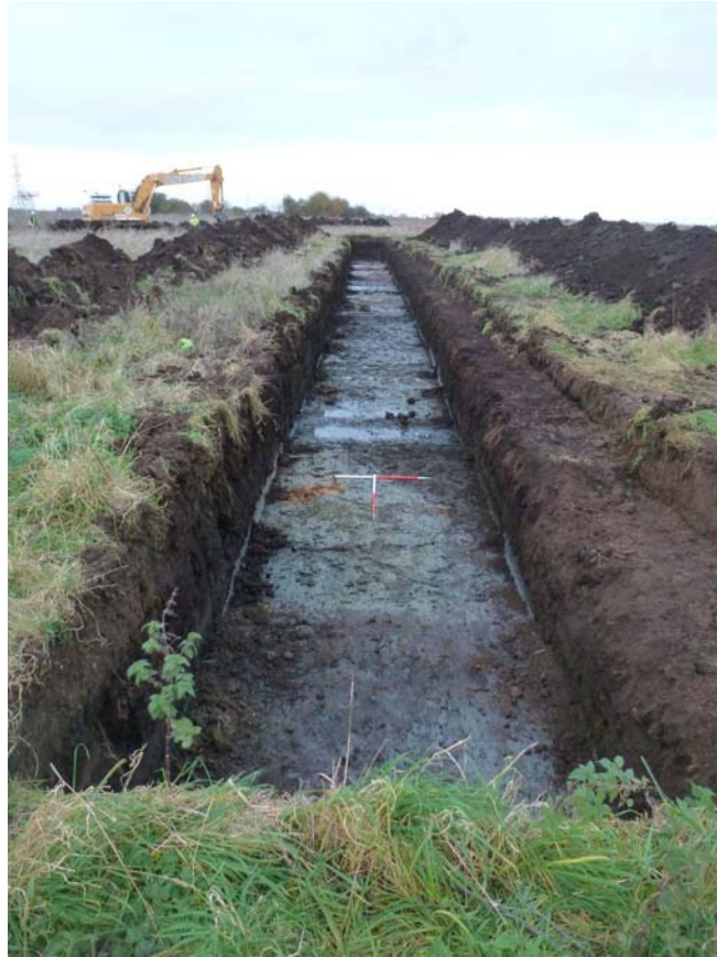
Trench 2, looking north-east Fig 3
