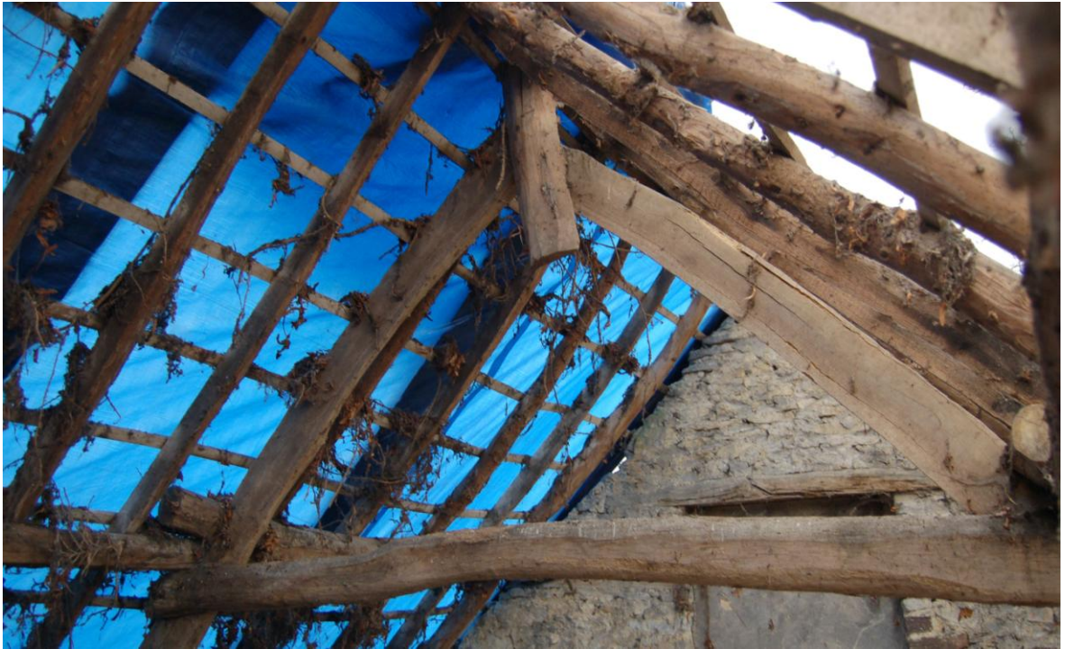
The collared truss, showing the wayney-edged timber, looking south
