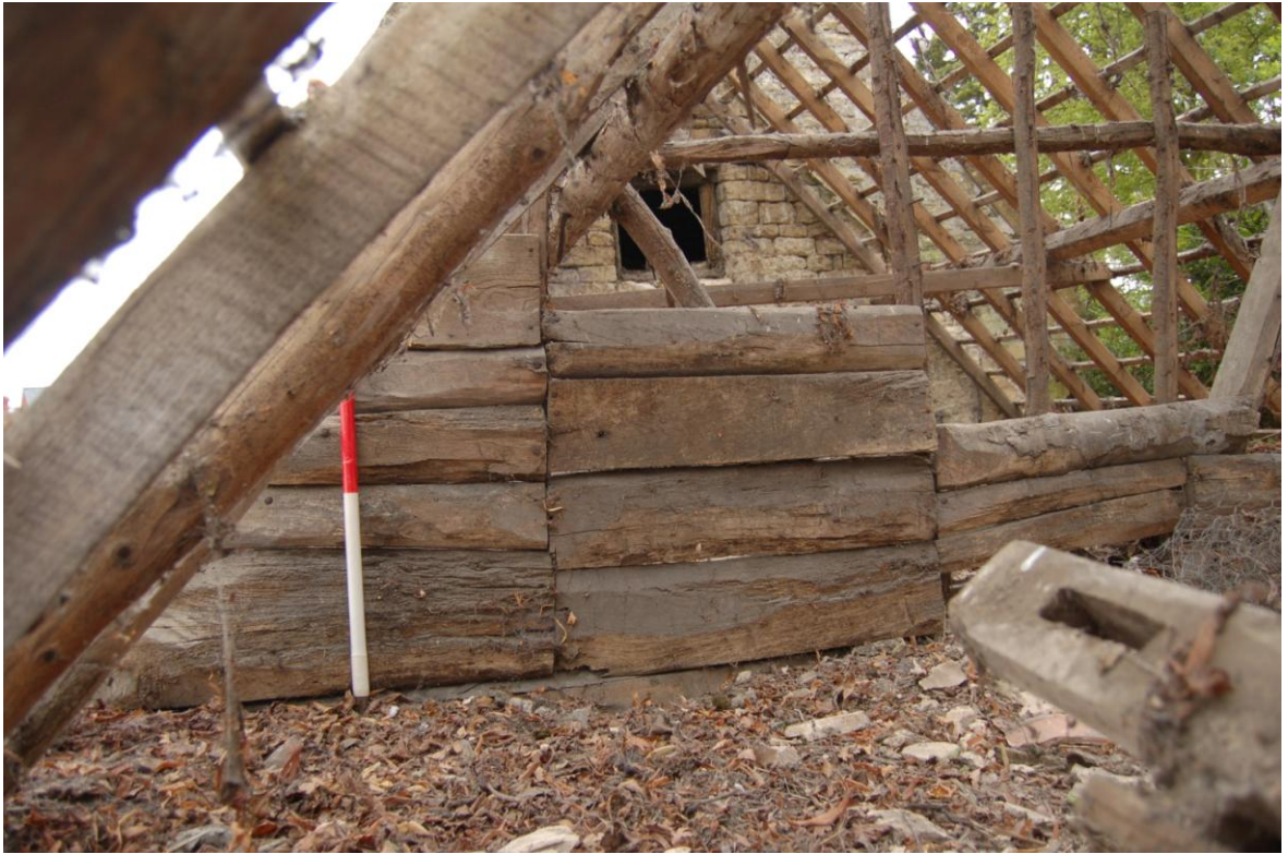
The partition again showing the wayne-edged nature of the timber
