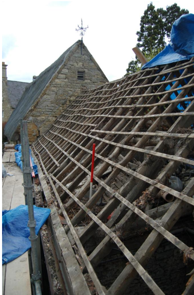
The roof, looking north-east, showing the battens still in place Fig 3
