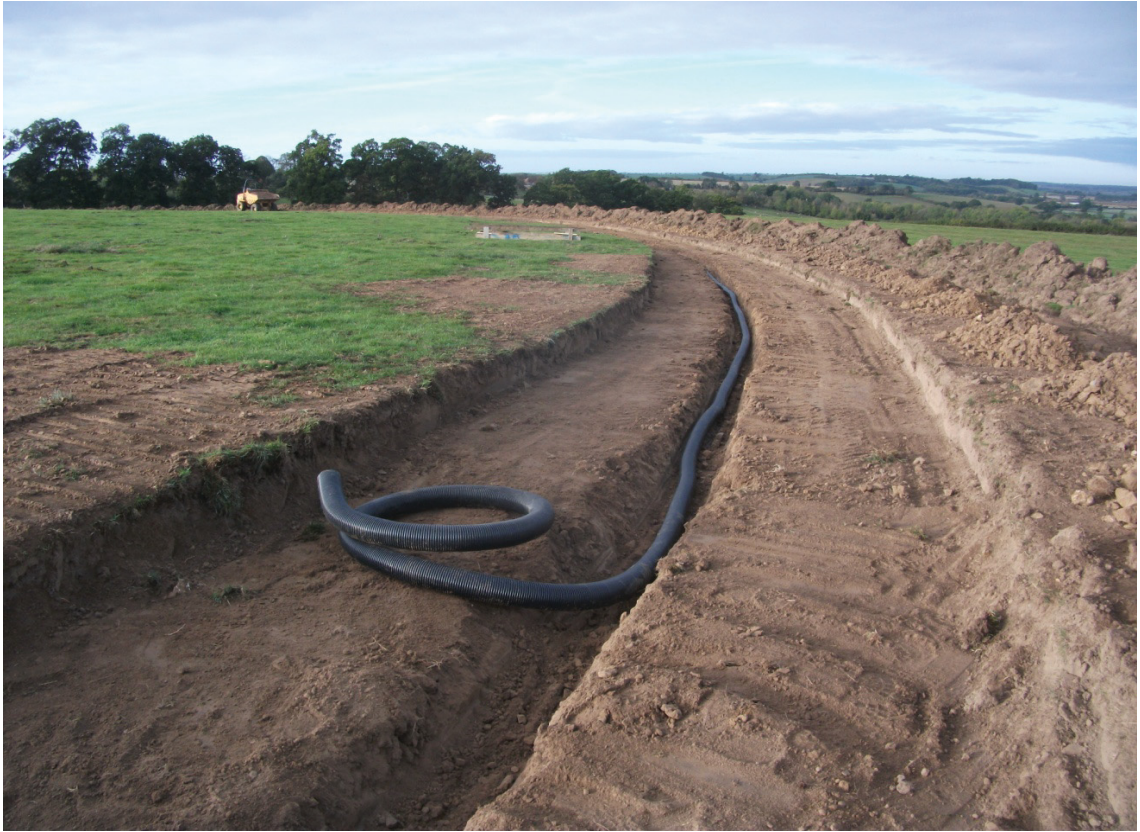
The laying of the drainage pipe, looking south-west Fig 6
