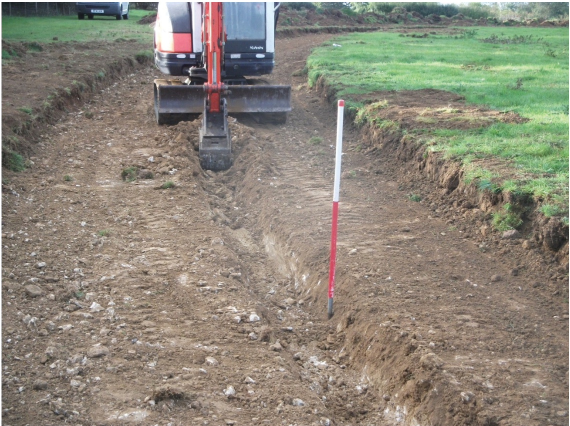
The excavation of the drainage trench, looking south-east Fig 5
