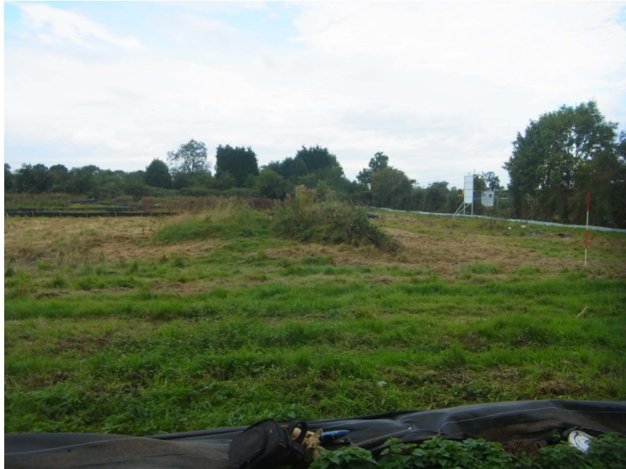
North-west corner of the development area prior to excavation
