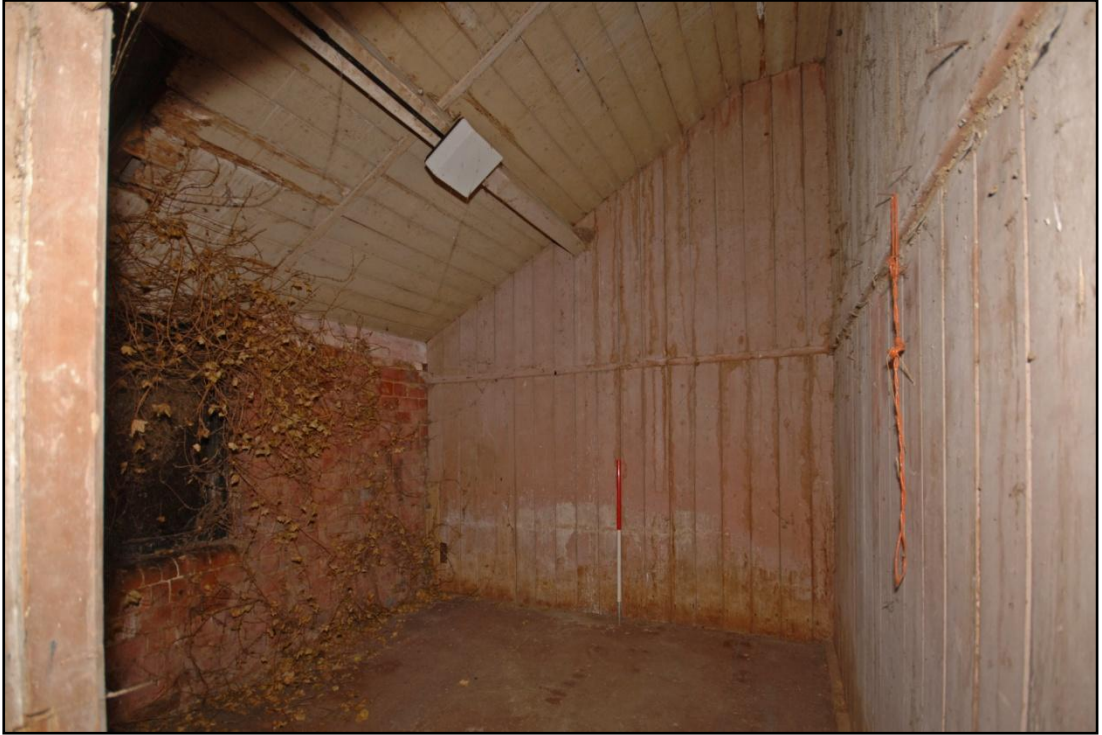
Tack Room 1, looking west Fig 19
