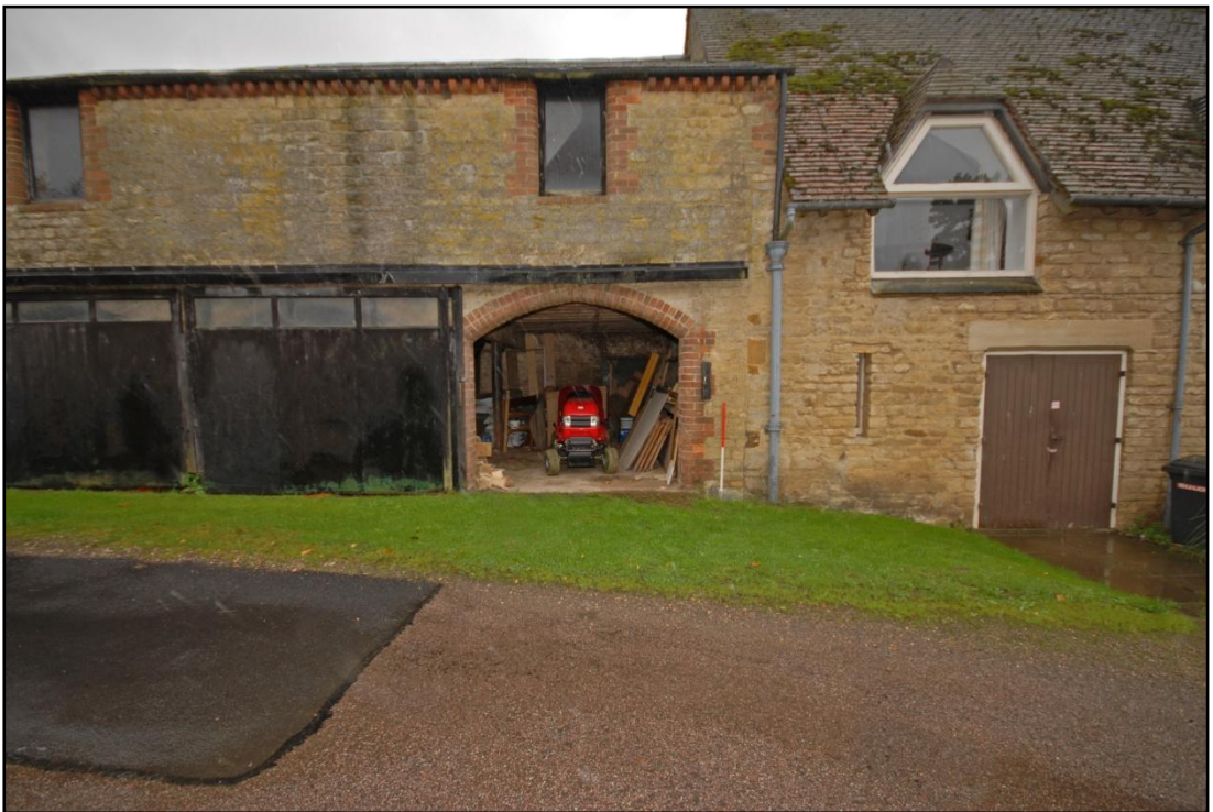
The north elevation of the barn, looking south Fig 10
