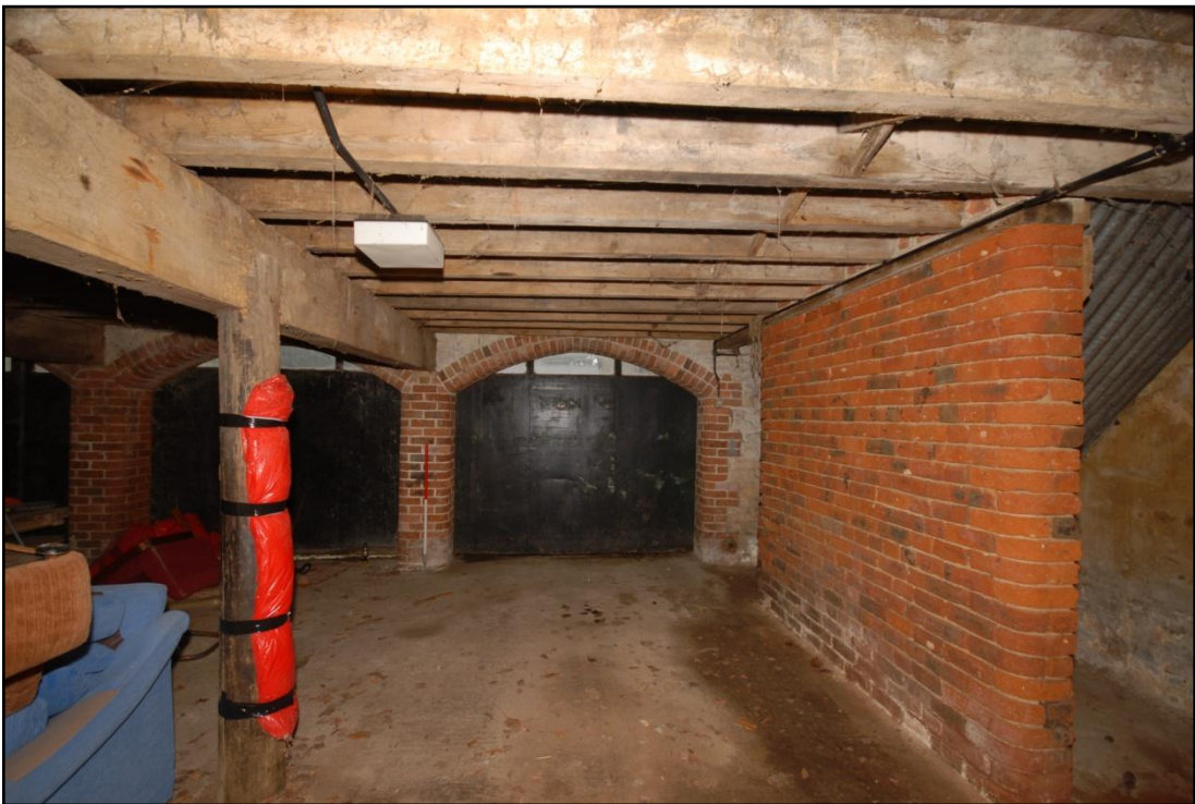
The ground floor, looking north with stairs to the right Fig 14
