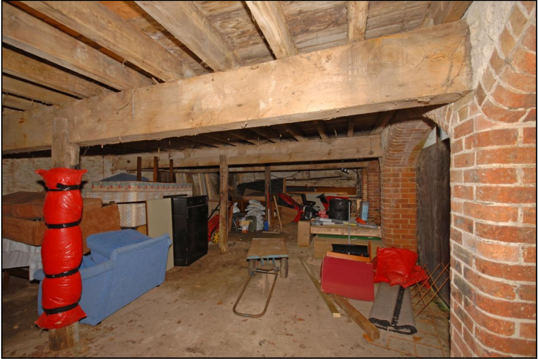
The ground floor, looking west Fig 13
