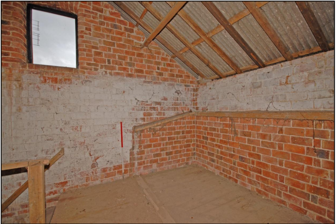
The first floor landing showing the scar of removed chicken coops to the right Fig 17
