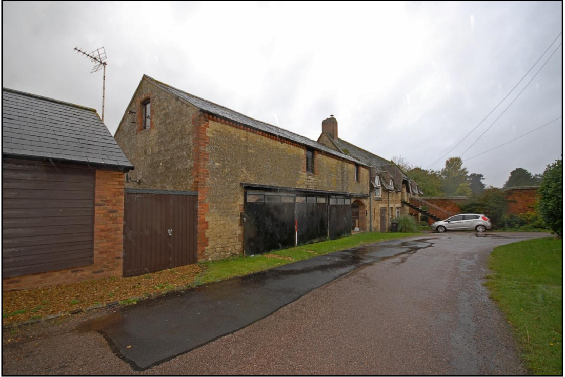
The north elevation of the Barn, looking west Fig 9
