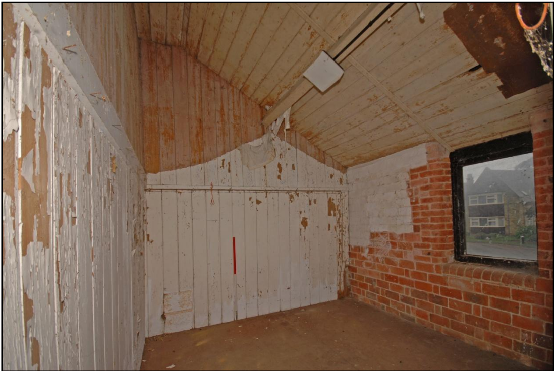
Tack Room 2, looking west Fig 20
