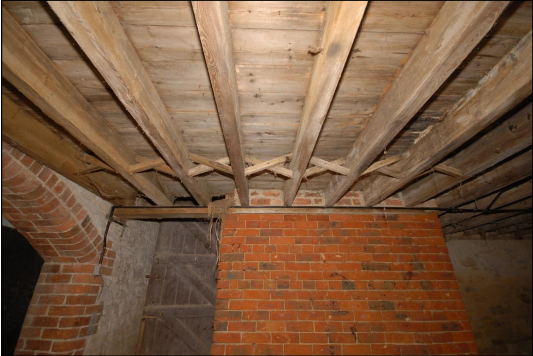
Detail of the roof structure with crossed bracing, looking east Fig 15
