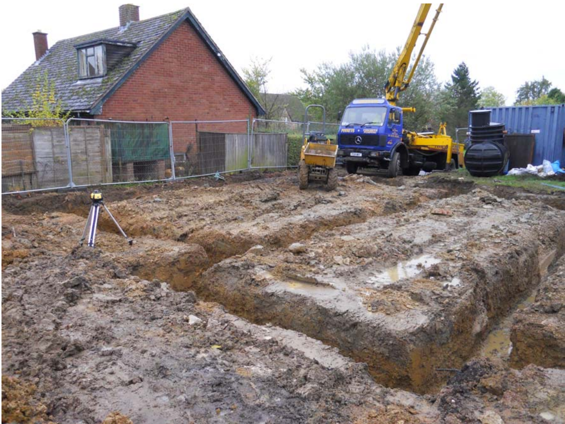
The foundation trenches, looking north
