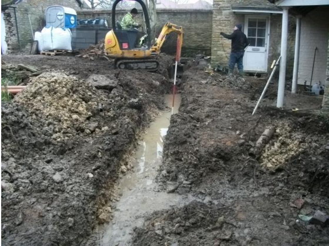
The excavation of the drainage trench Fig 26
