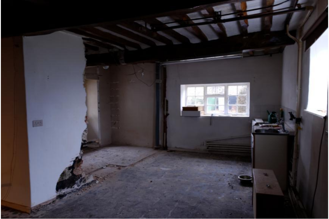
Room 5, the kitchen subsequent to demolition of a dividing wall Fig 17
