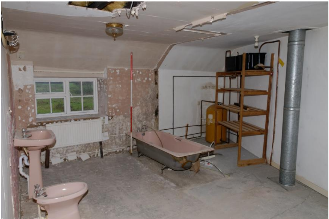
Room 10, subsequent to the demolition of the dividing walls Fig 22
