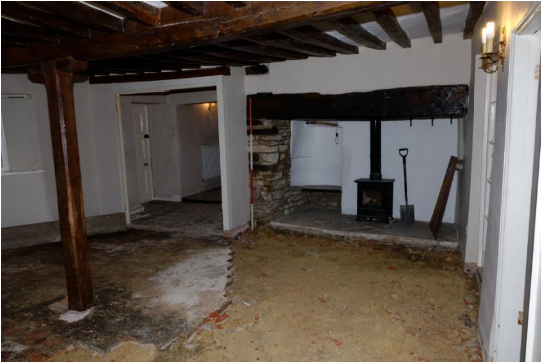
Room 2, floor partially lifted prior to survey Fig 13
