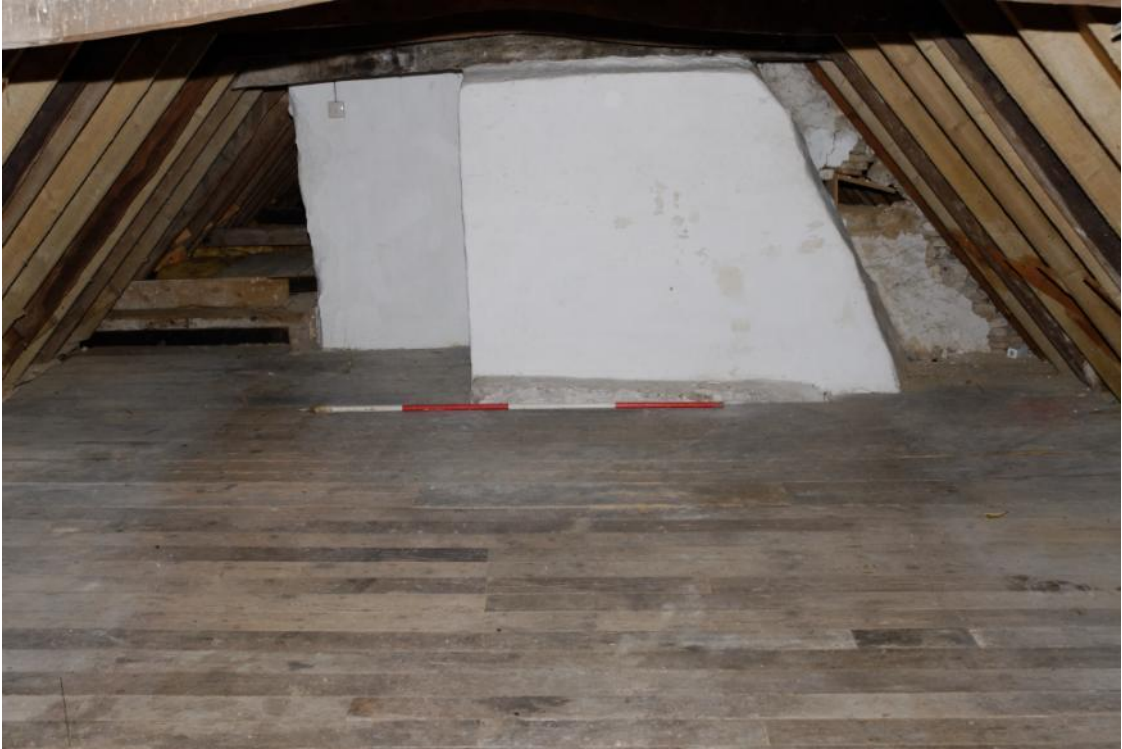
The attic, Room 11 Fig 23
