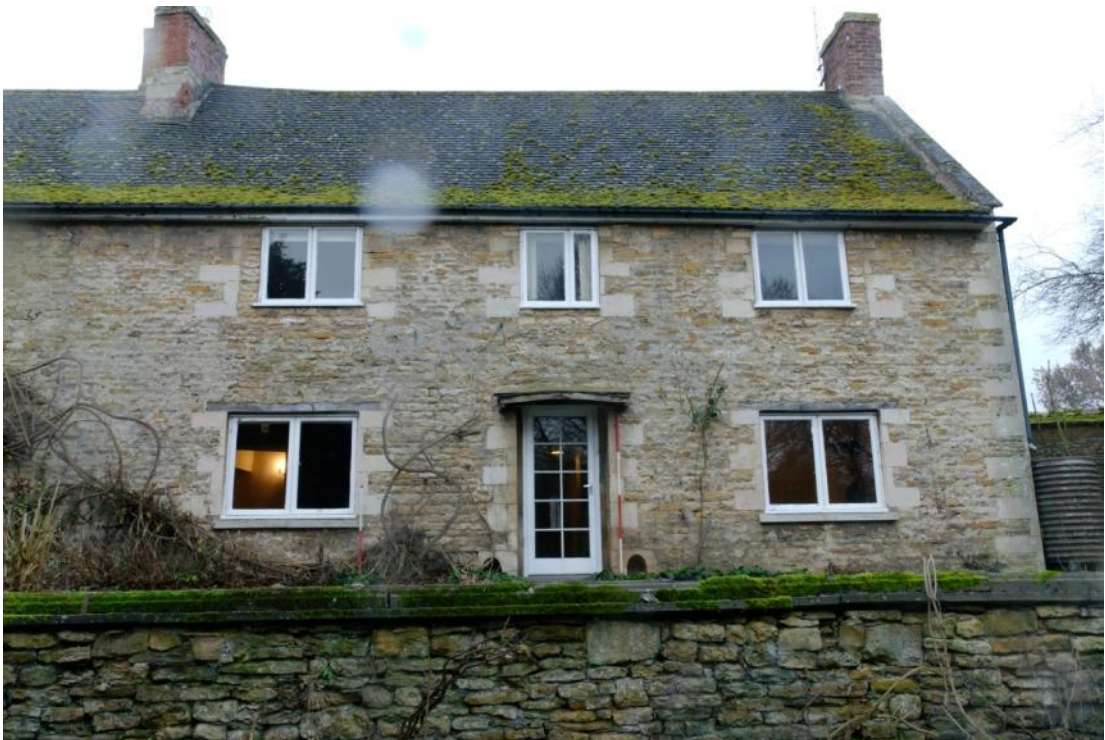
The rear south-east facing elevation of the building Fig 7
