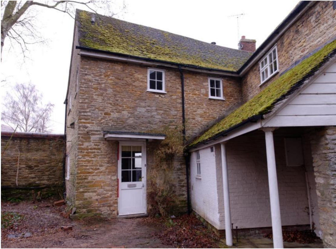
The porch, looking north-east Fig 10
