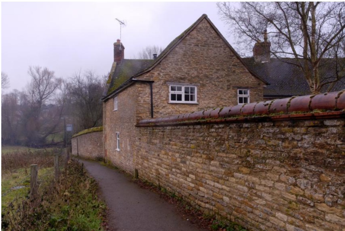
The north-east facing elevation, looking down the public footpath Fig 5
