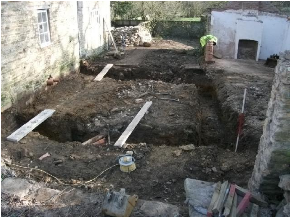
General view of the foundation trenches, looking south-east Fig 24
