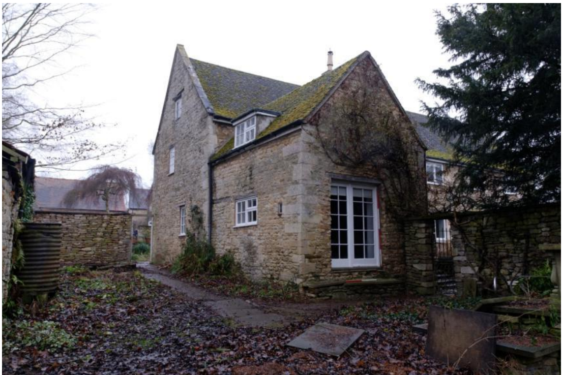
The French window in the south facing gable, looking north Fig 9
