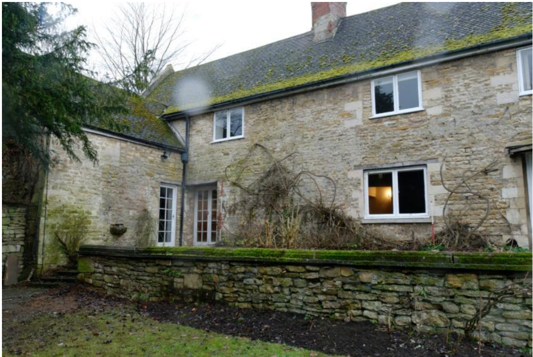
The rear south-east facing elevation of the building, looking west Fig 8
