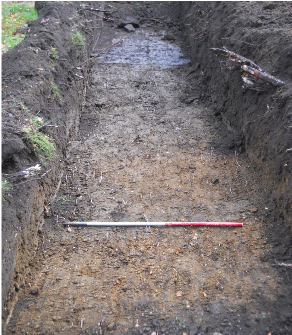
Trench 1, south-west end showing edge of pond Fig 4
