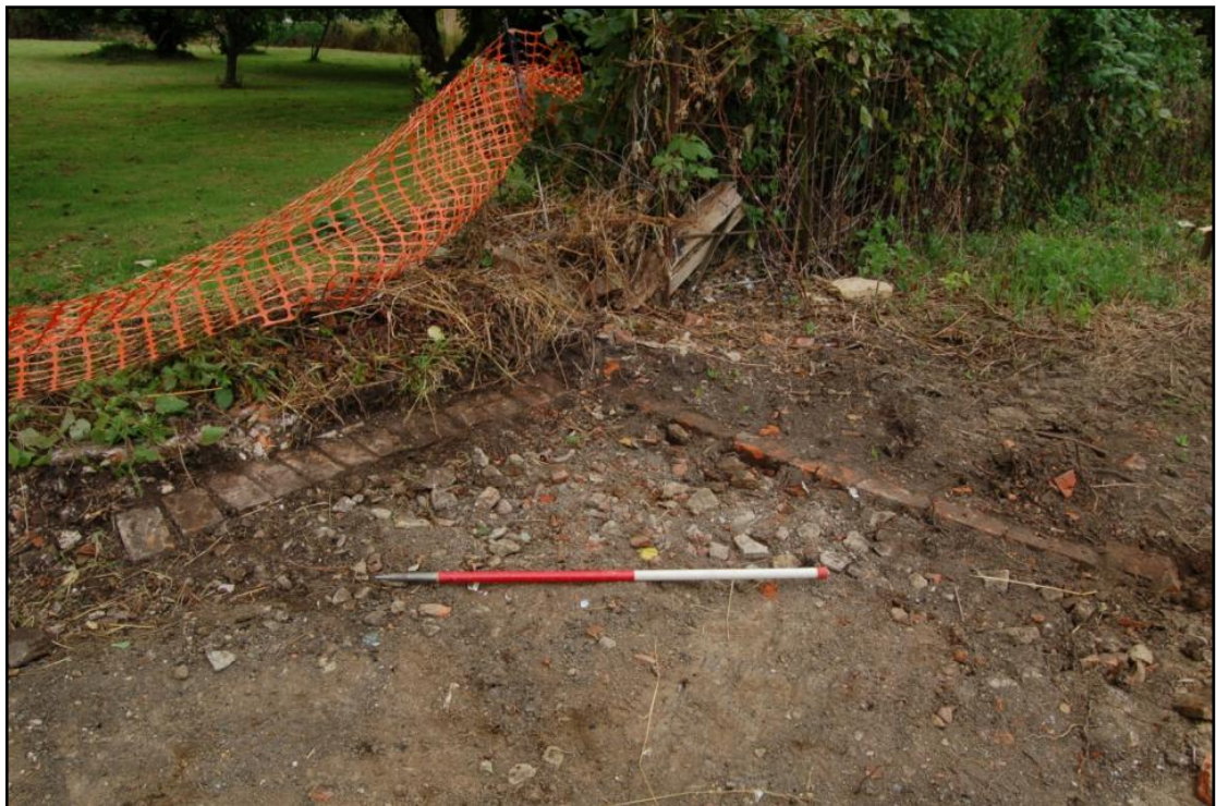
The brick foundations of Room 4, looking north-west Fig 9
