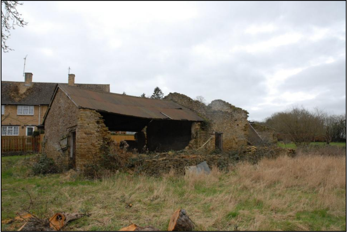
General view of the site prior to demolition of the outbuildings, looking south-west Fig 20
