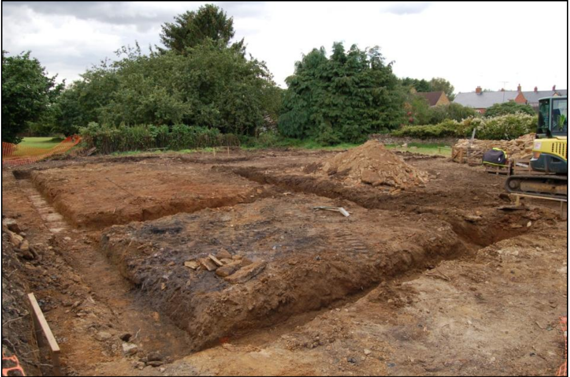
General view of the excavated footings, looking north-west Fig 18
