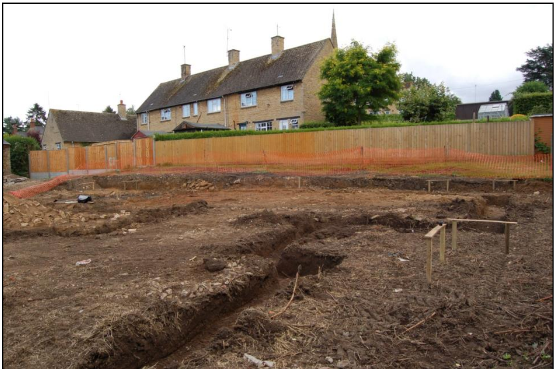
General view of the excavated footings, looking south Fig 19
