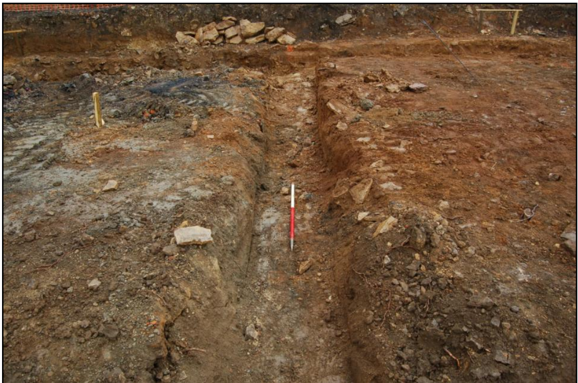
The central footings, looking south Fig 15
