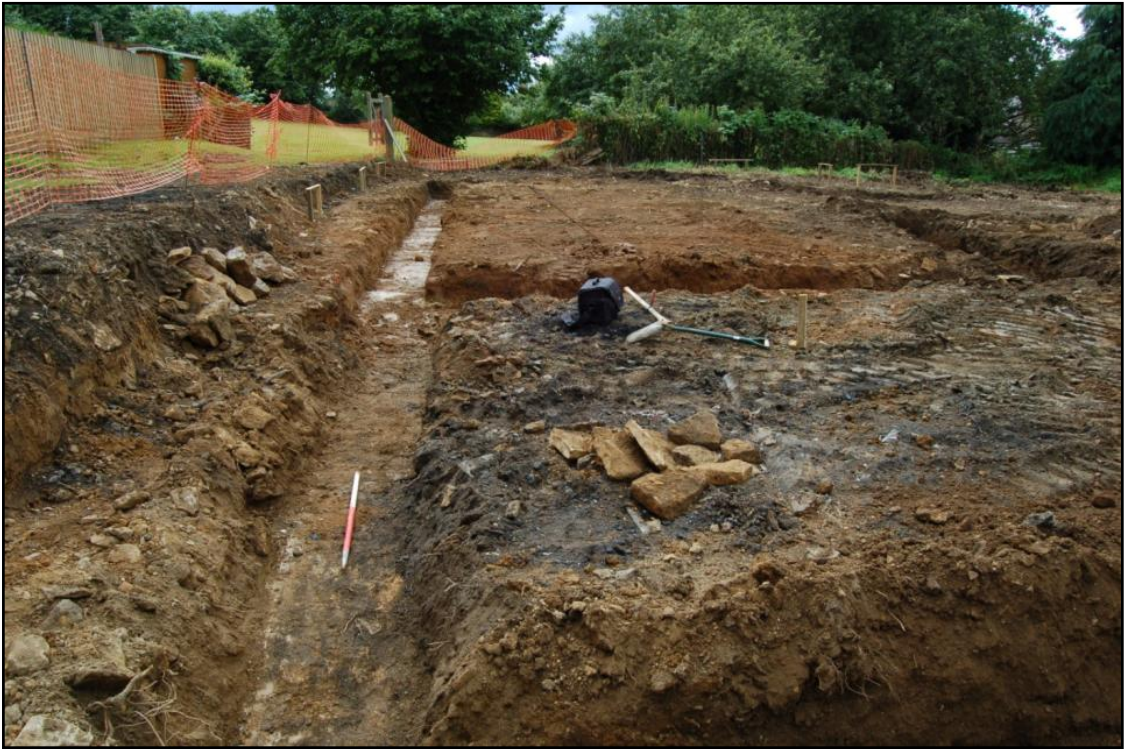
The southern footings, looking west Fig 16
