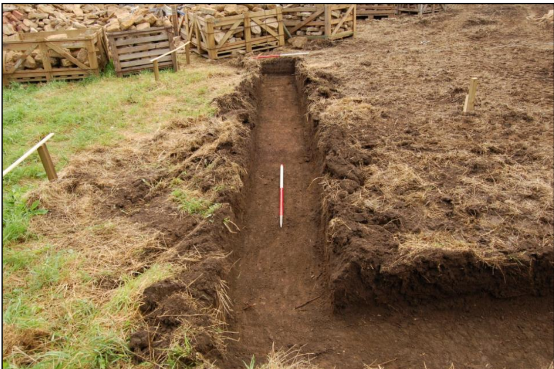
The northern footings, looking east Fig 5
