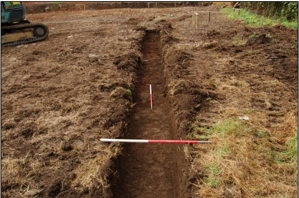
The northern footings, looking south Fig 7
