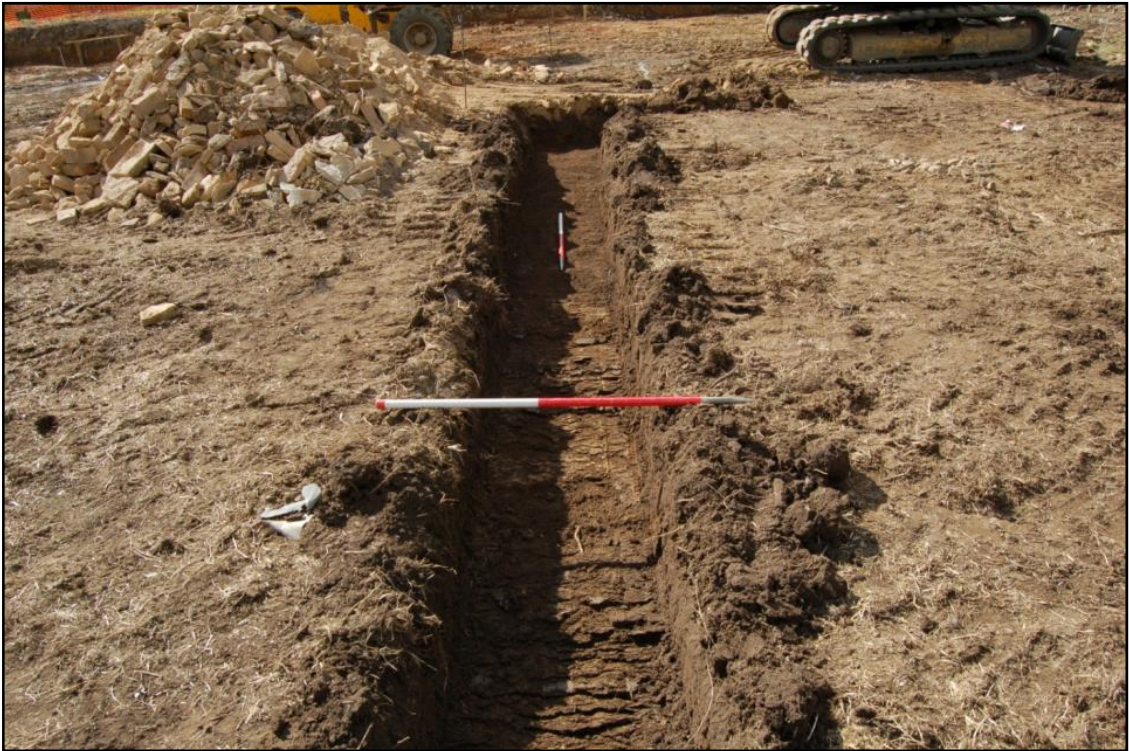
The northern footings, looking south Fig 6
