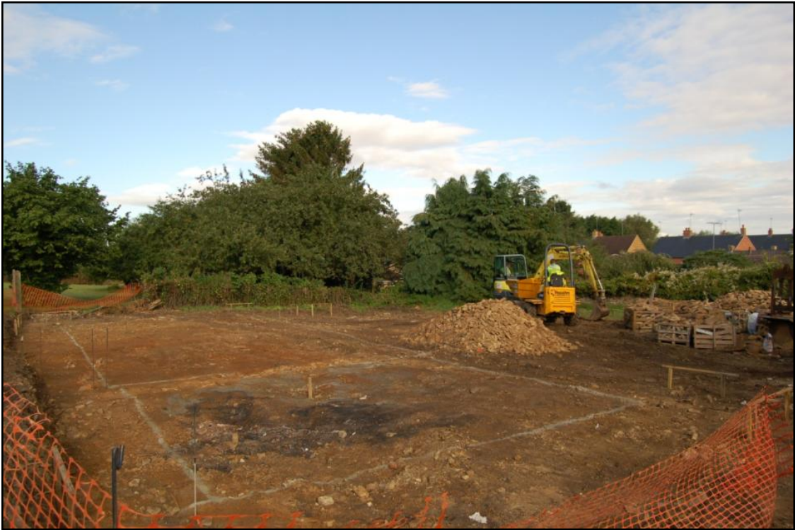
The site prior to excavation of the footings Fig 4
