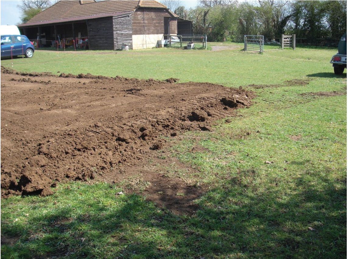
Building up the southern half of the area, looking north-east Fig 5
