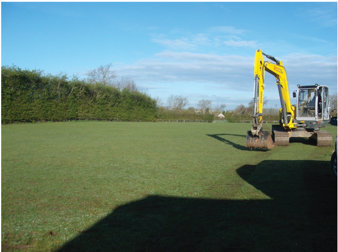
The investigation area, looking north-west Fig 3
