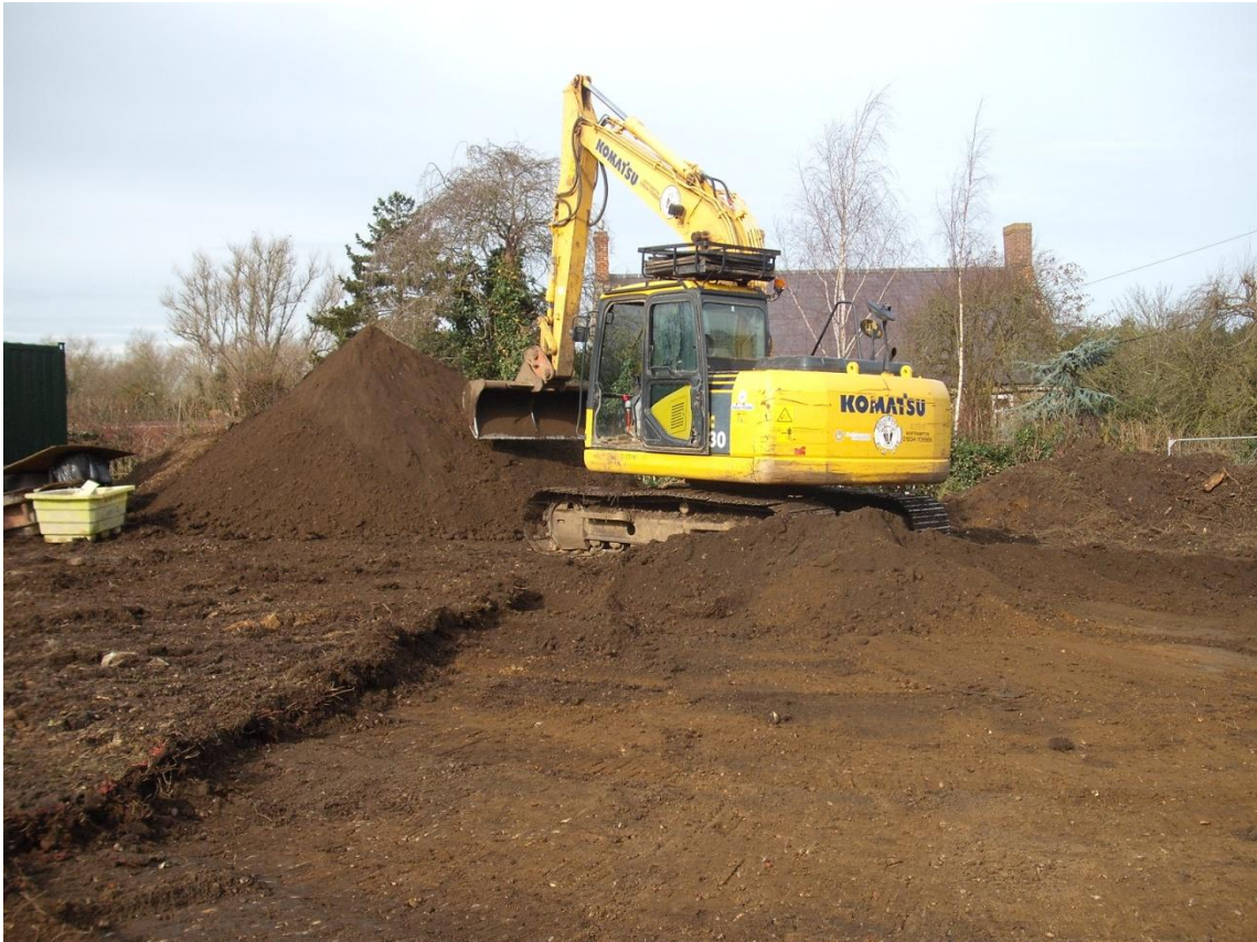
The groundworks in progress, looking north-west Fig 5
