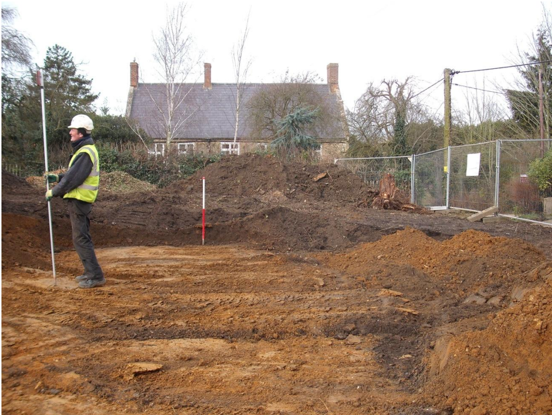
Reduction of the area to formation level, looking north-west Fig 6
