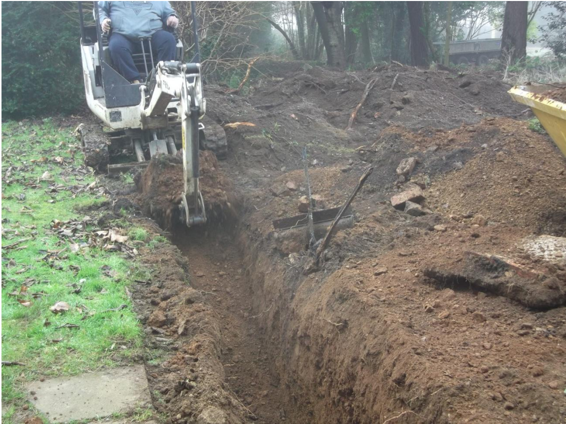
General view of the groundworks in progress, looking south Fig 5
