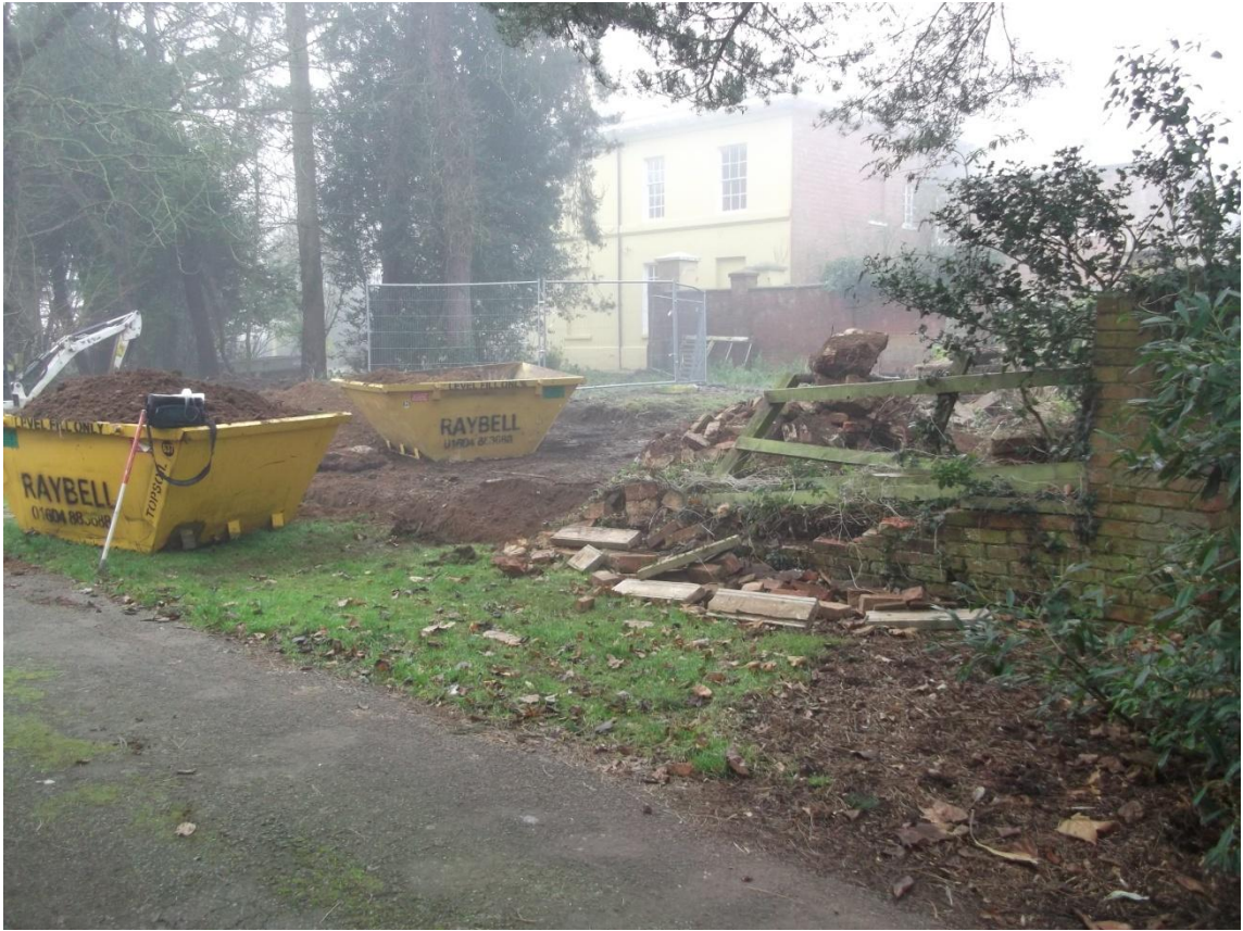
The opening created in the boundary wall, looking west Fig 4
