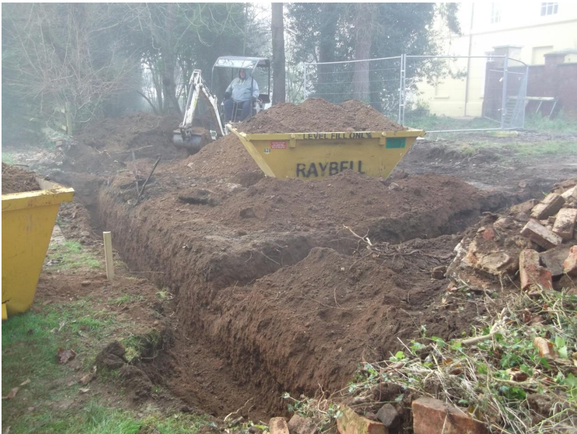
General view of the foundation trenches, looking south-west Fig 6
