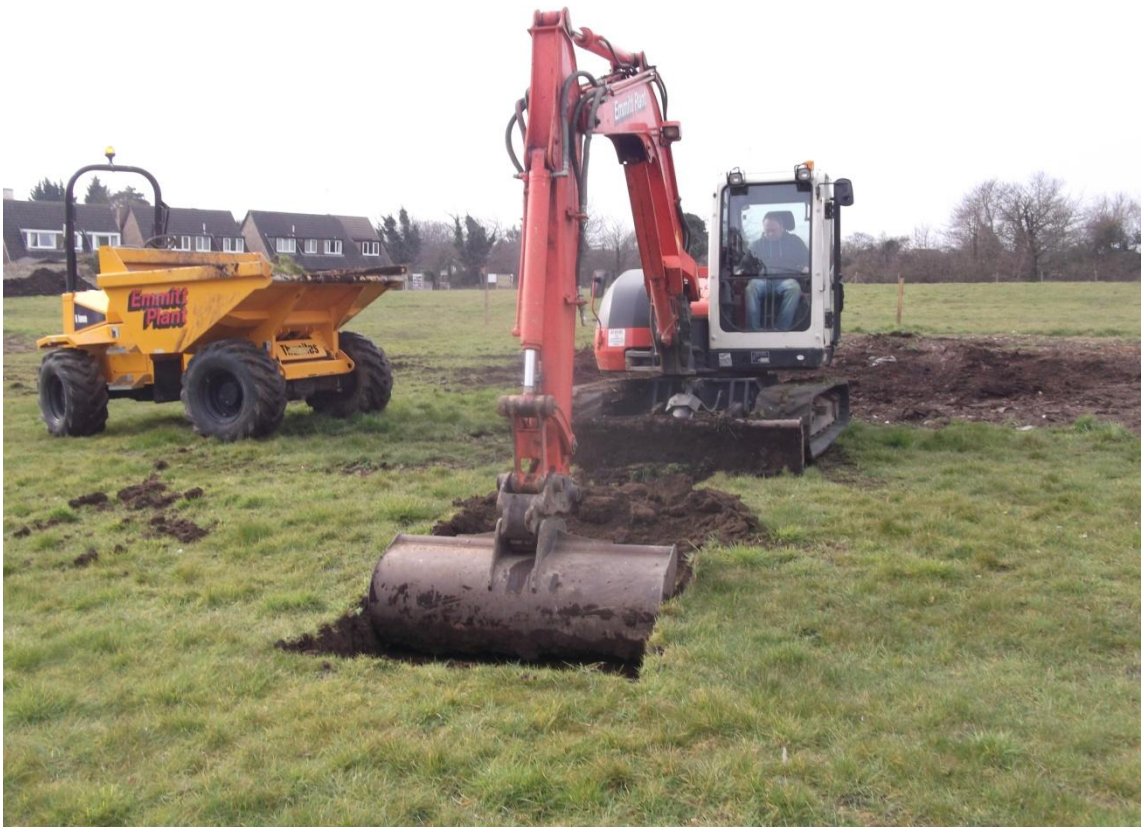
General view of the groundworks, looking south-east Fig 4
