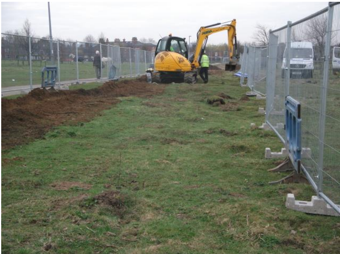
The groundworks in progress, looking south Fig 4
