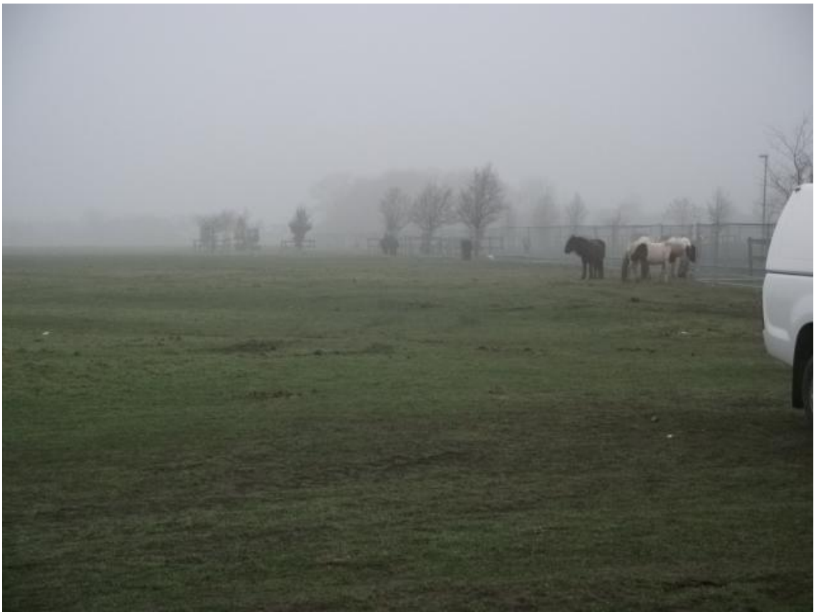
The pipeline route prior to the start of groundworks, looking north-west Fig 3
