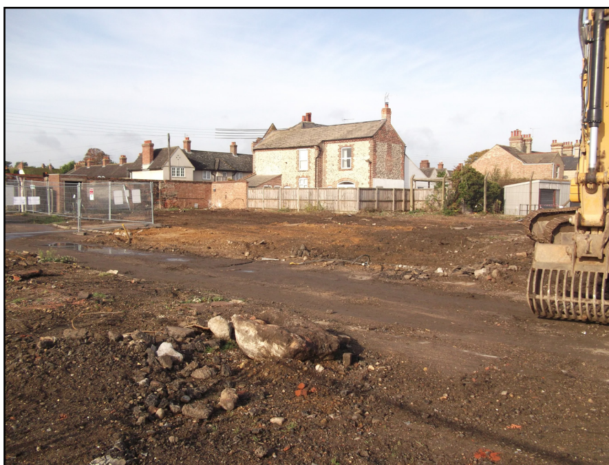
Investigation area, looking south-west
