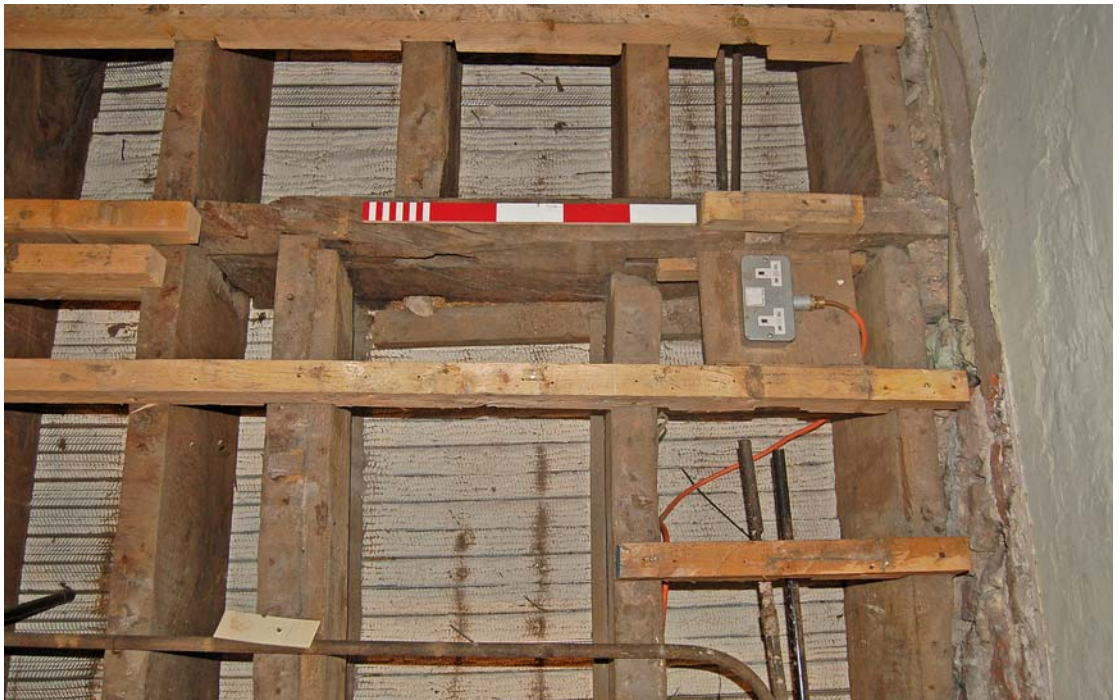
Fig 14: First floor south-west corner position of former stair or hatch
