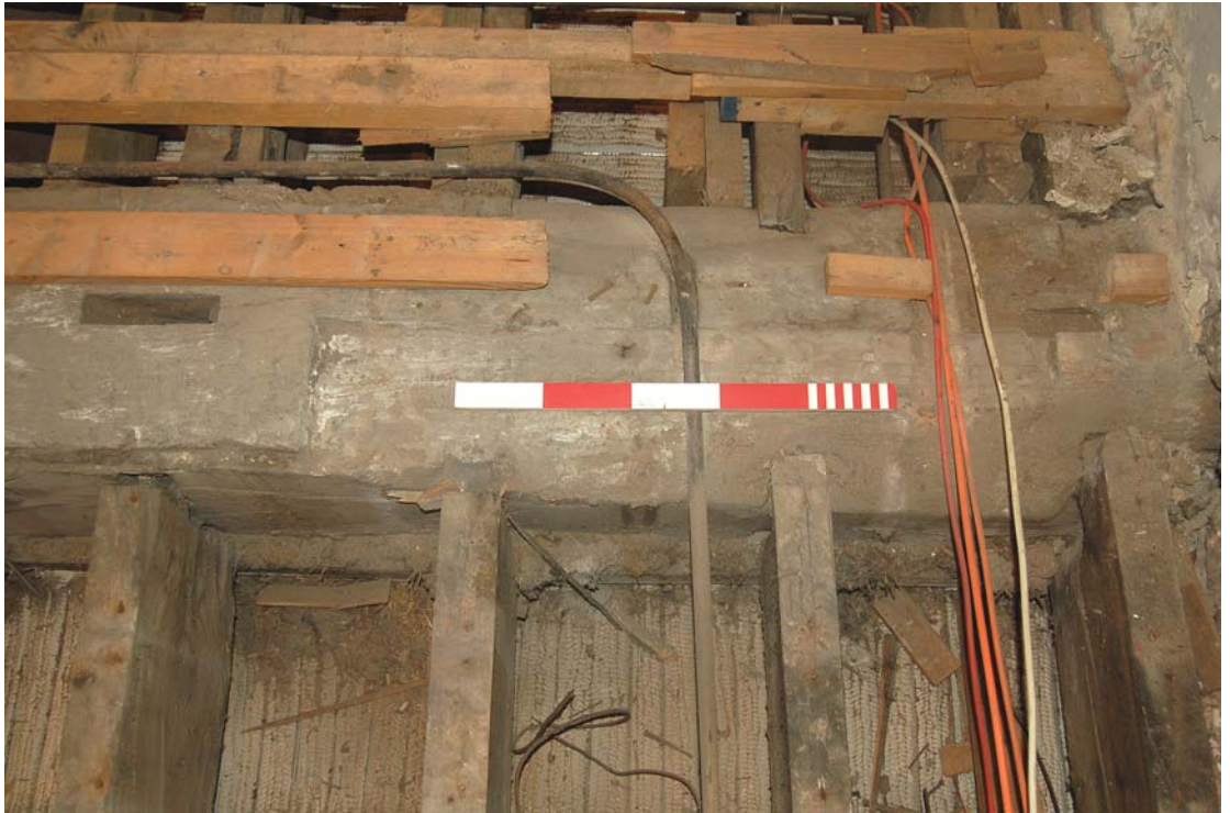
Fig 10: First floor mortice for doorway in partition on beam C
