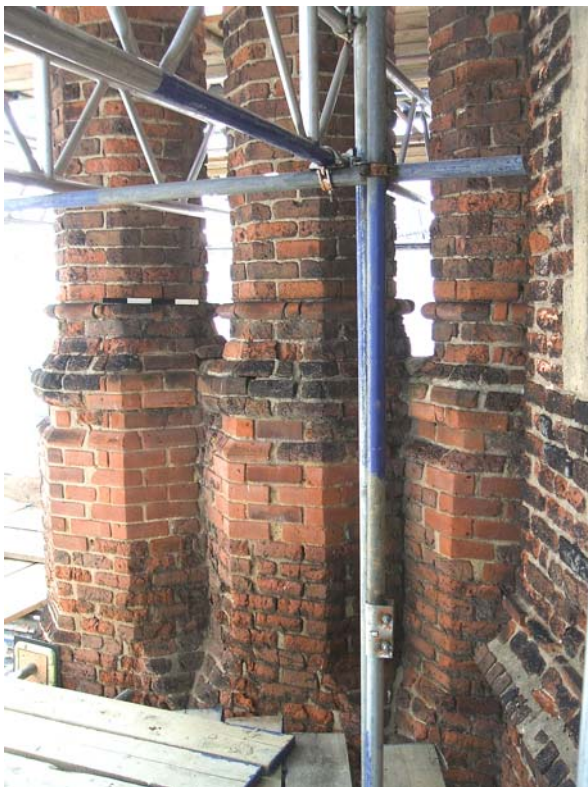
Fig 26: General view of lower part of chimney looking west
