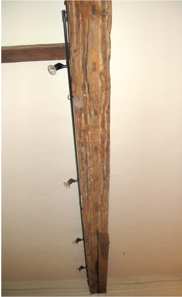
Fig 11: First floor beam above beam C showing corresponding slots for partition
