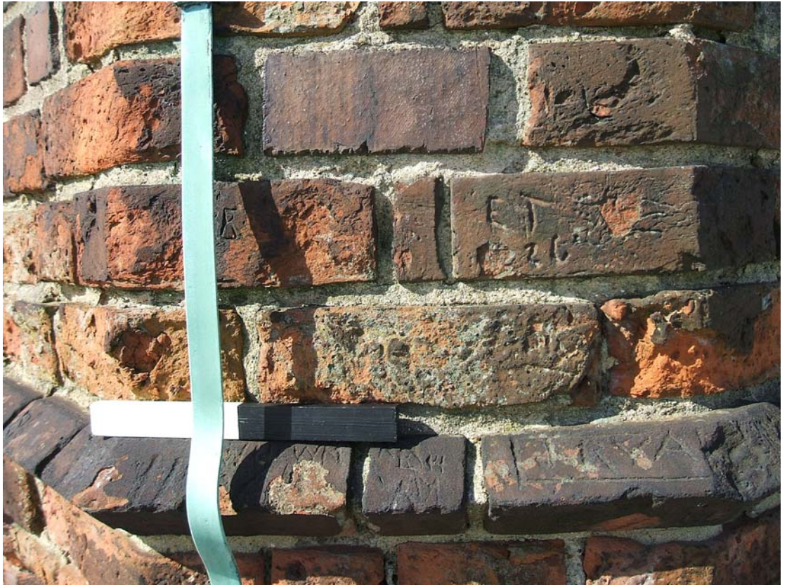
Fig 23: Graffiti on north chimney stack
