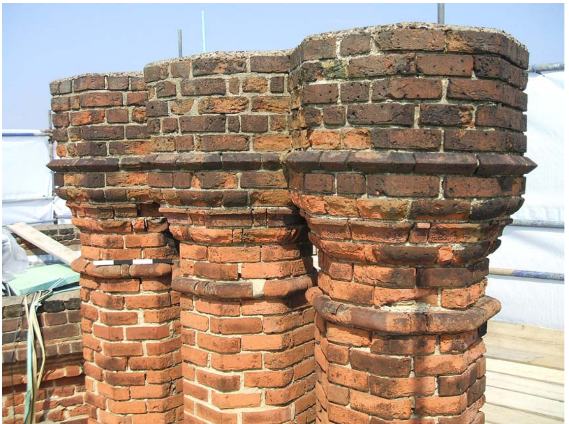
Fig 24: General view of chimney looking north-east
