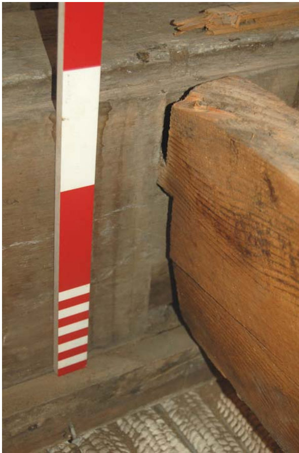
Fig 16: First floor Pine joist set into oak beam
