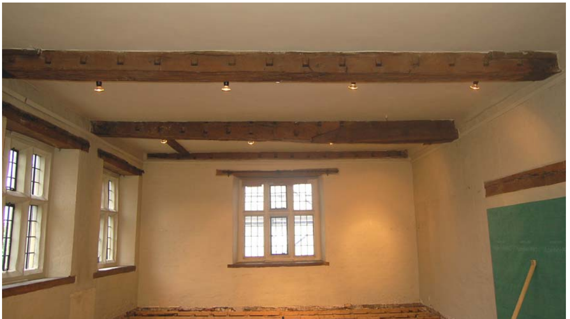
Fig 12: First floor general view of beams
