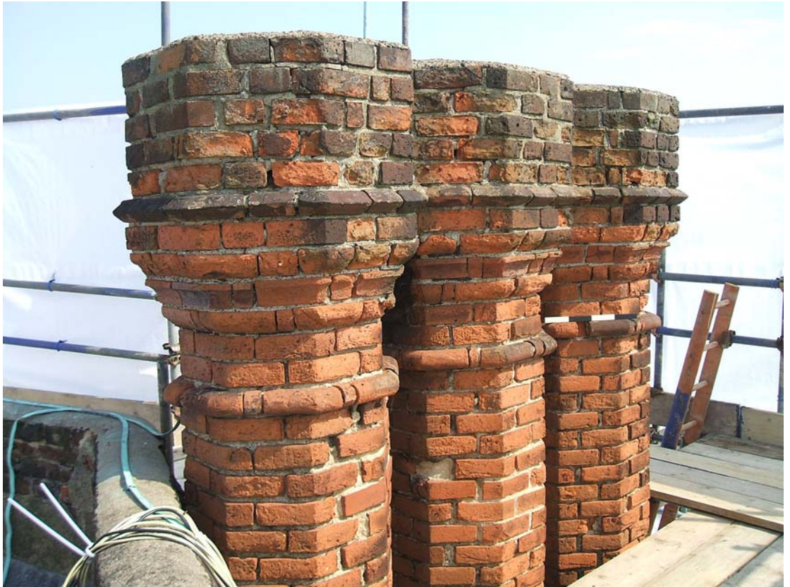
Fig 25: General view of chimney looking south-east
