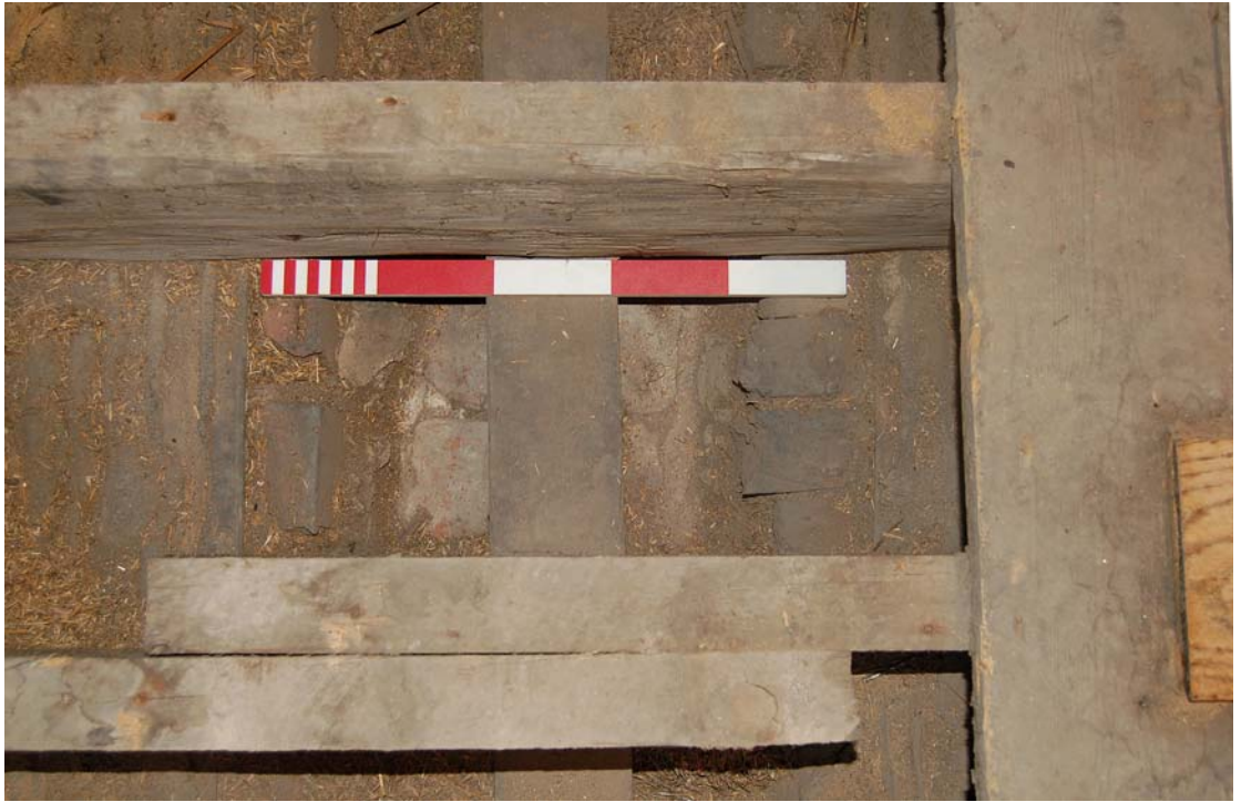
Fig 15: First floor top of wall below joists
