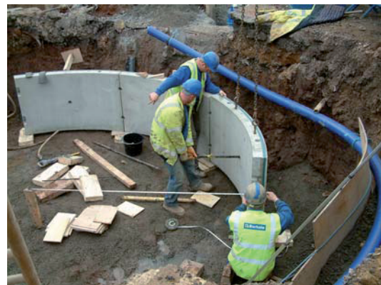
Plate 10: Constructing concrete shaft.
