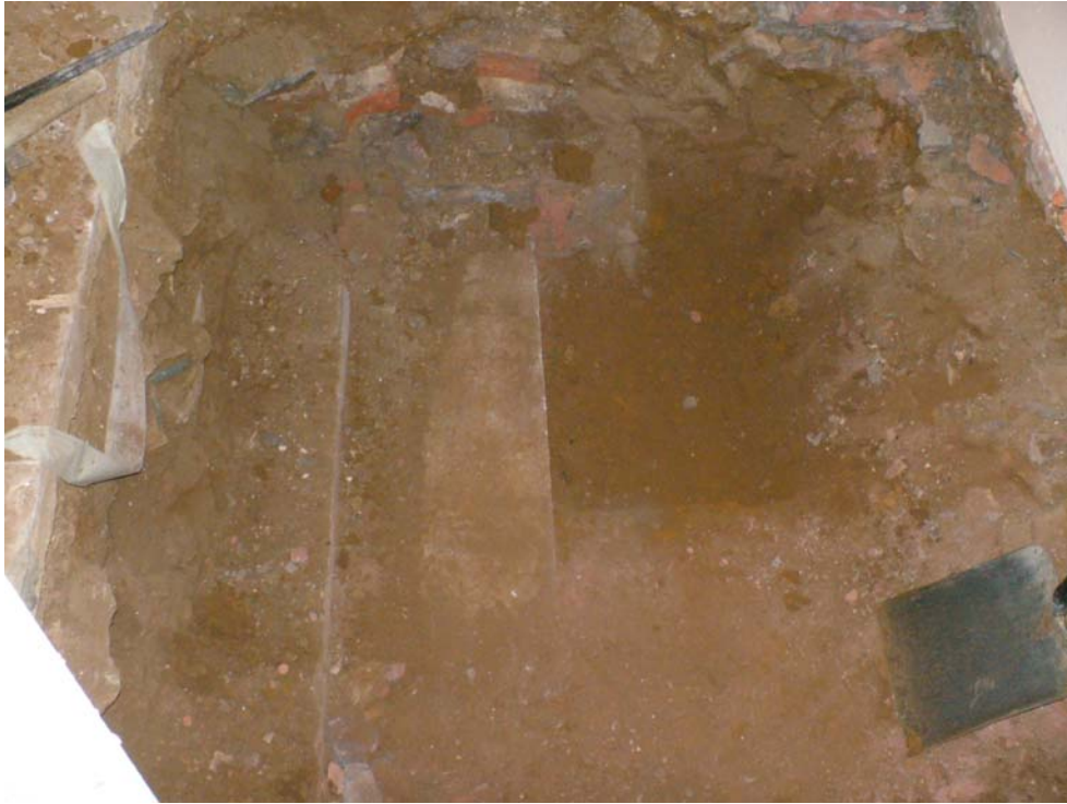
Plate 1 Lift installation pit showing concrete raft and rubble
