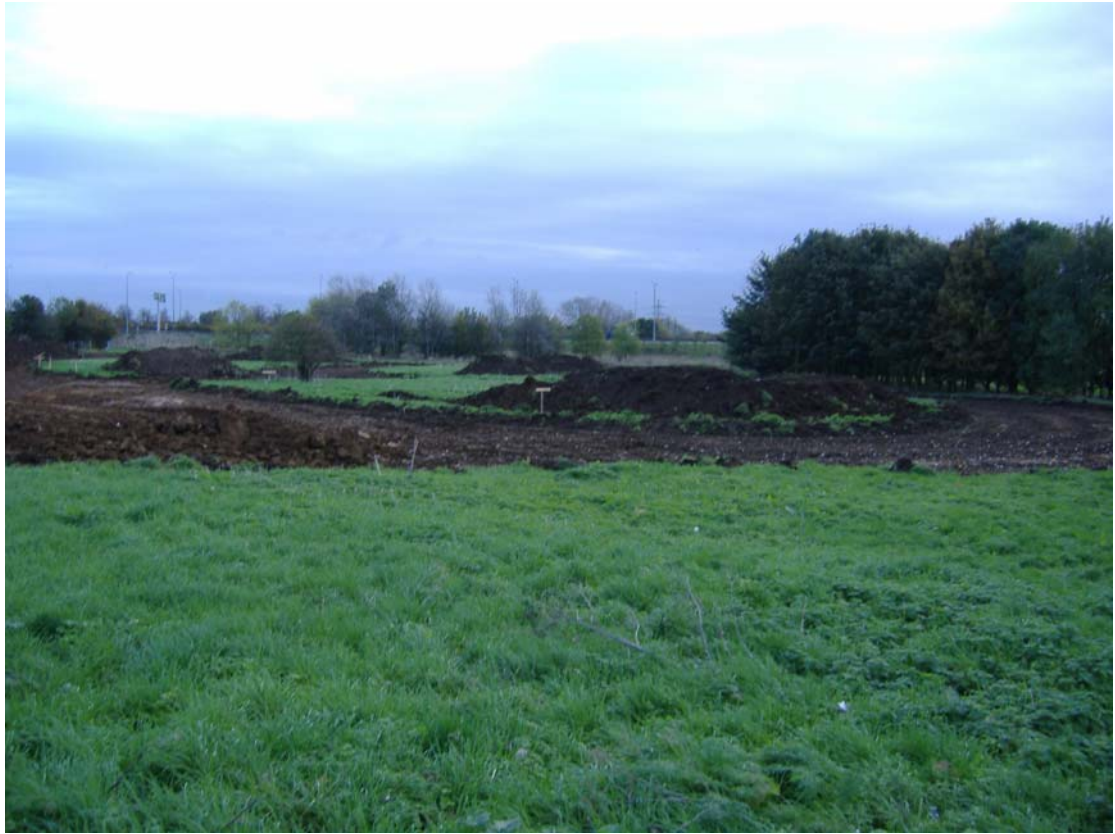
Plate 3 Overview of ground works, looking north-west
