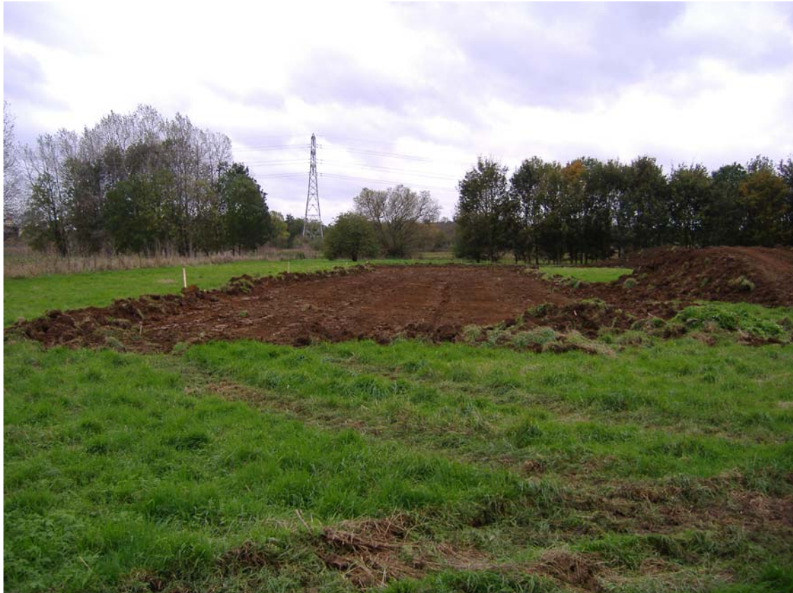
Plate 1 Topsoil stripping, looking north
