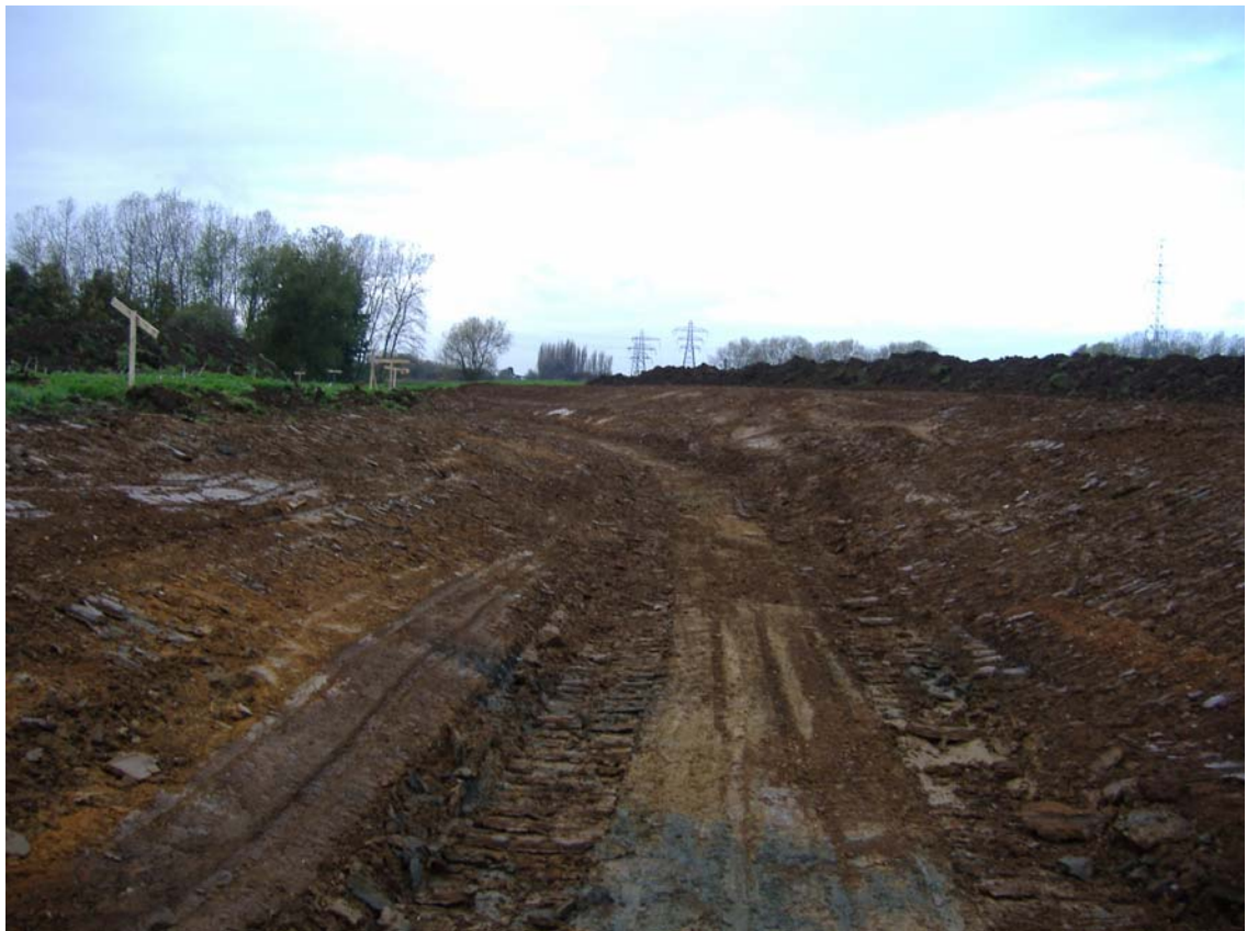
Plate 2 Depth of excavation, looking north-east
