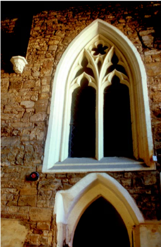
Plate 4: Window in south wall of chapel, showing previous embrasure in wall.
