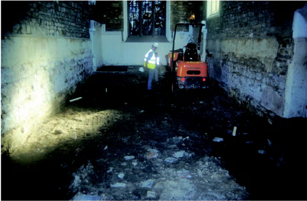
Plate 1: The works of conversion, interior of chapel.
