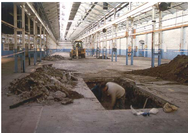
Plate 10: Excavating within main works
