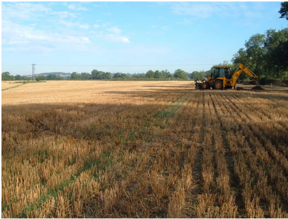
Plate 1: Excavating Trench 2 at the south end of road corridor, looking north-west
