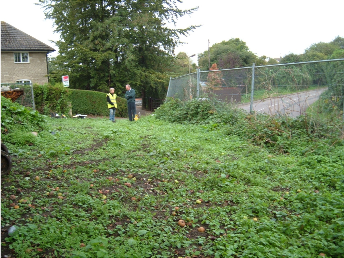
Plate 1: Site prior to excavation, facing west.
