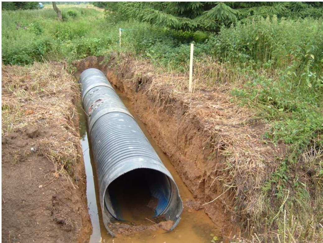
Plate 4: Drainage works to north-west of mill, looking west
