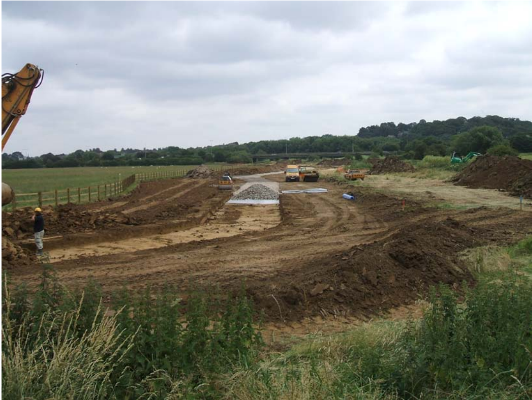
Plate 1: Haul road construction, looking east
