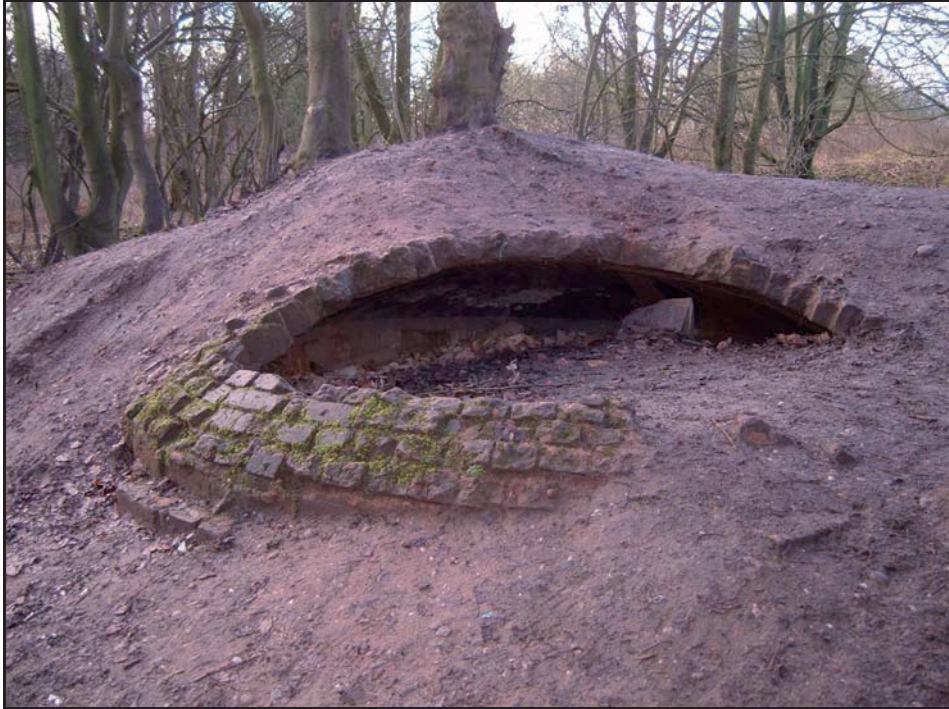
Plate 1 The ice house looking south prior to cleaning
