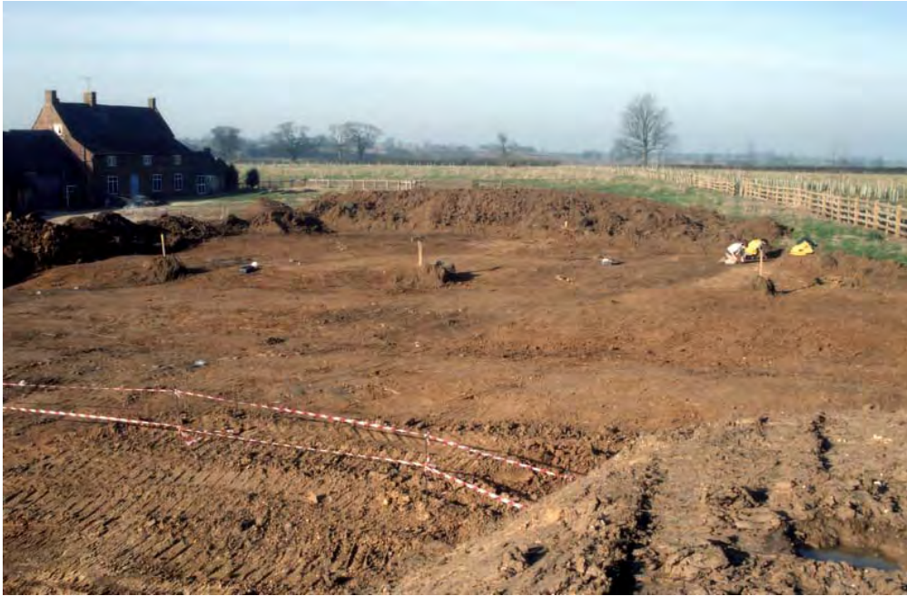
Plate 1: Site prior to excavation
