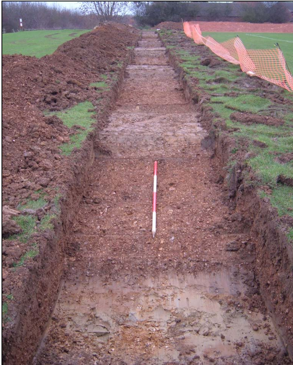
Plate 1: Example of excavated trench from Gunthorpe playing fields
