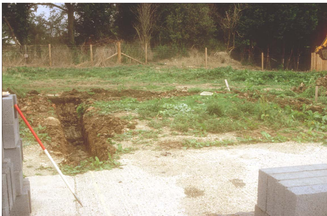
Plate 2: Ground-works in progress, with the moat bank in the background
