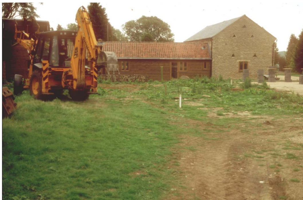
Plate 1: The area of development at the start of ground-works
