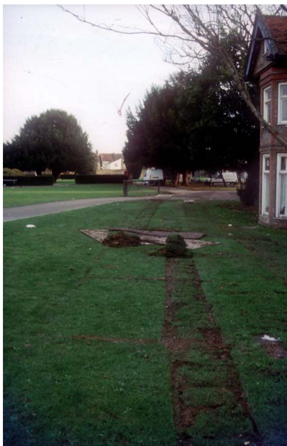
Plate 2: General view of the line the service trench
