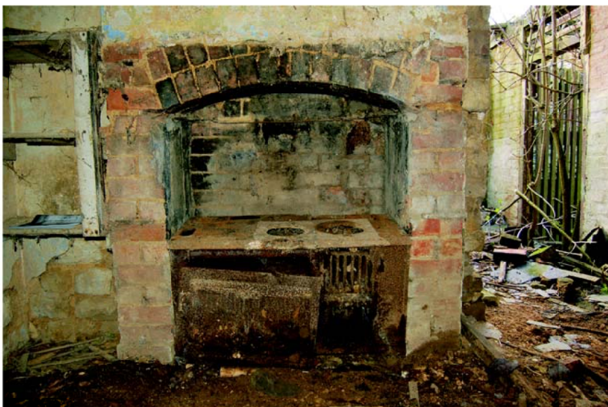
Plate 7: Cast iron cooking stove in Room 1, looking north.
