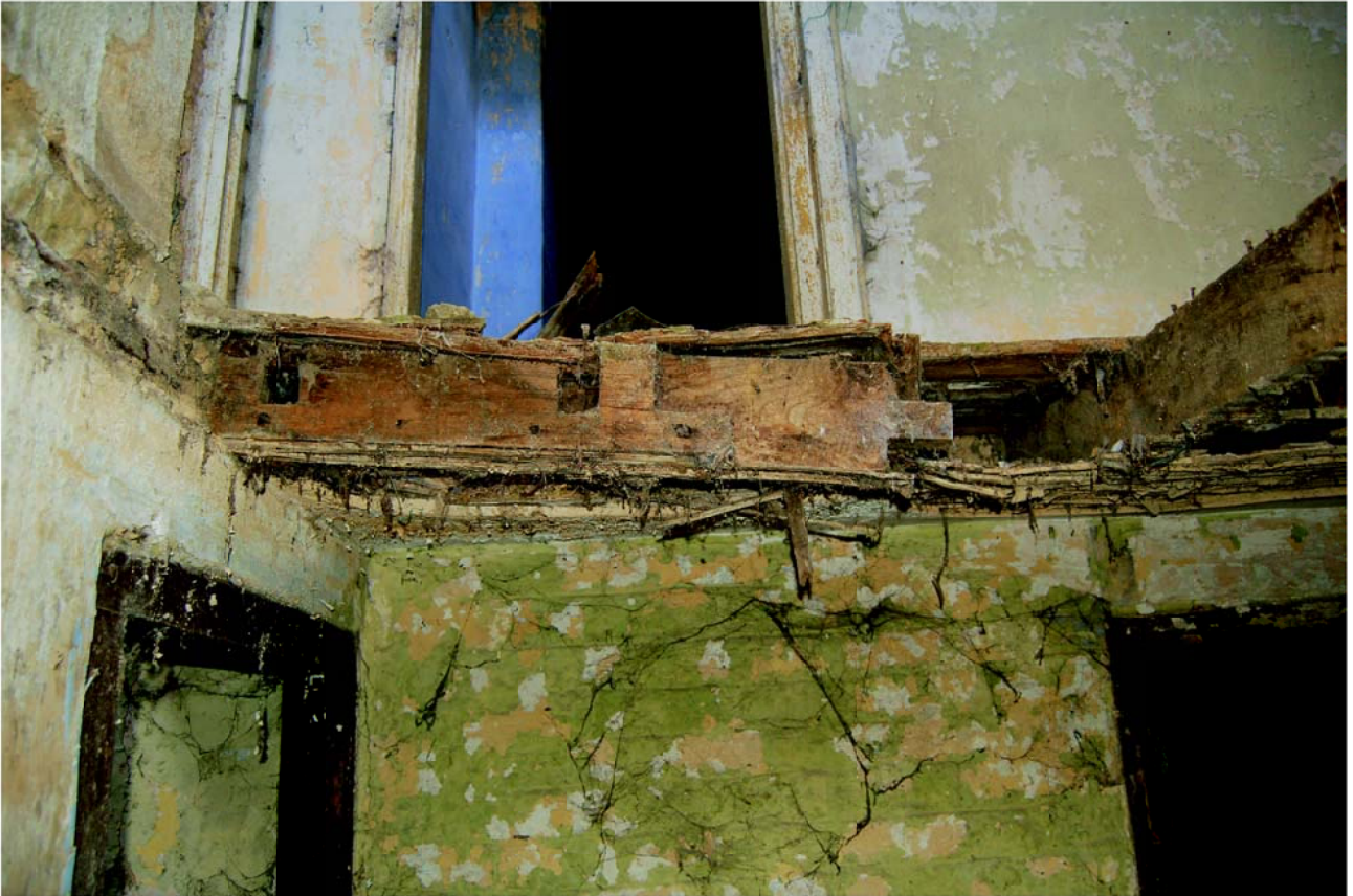
Plate 8: Trimmer at top of former stairs in western cottage, looking south.
