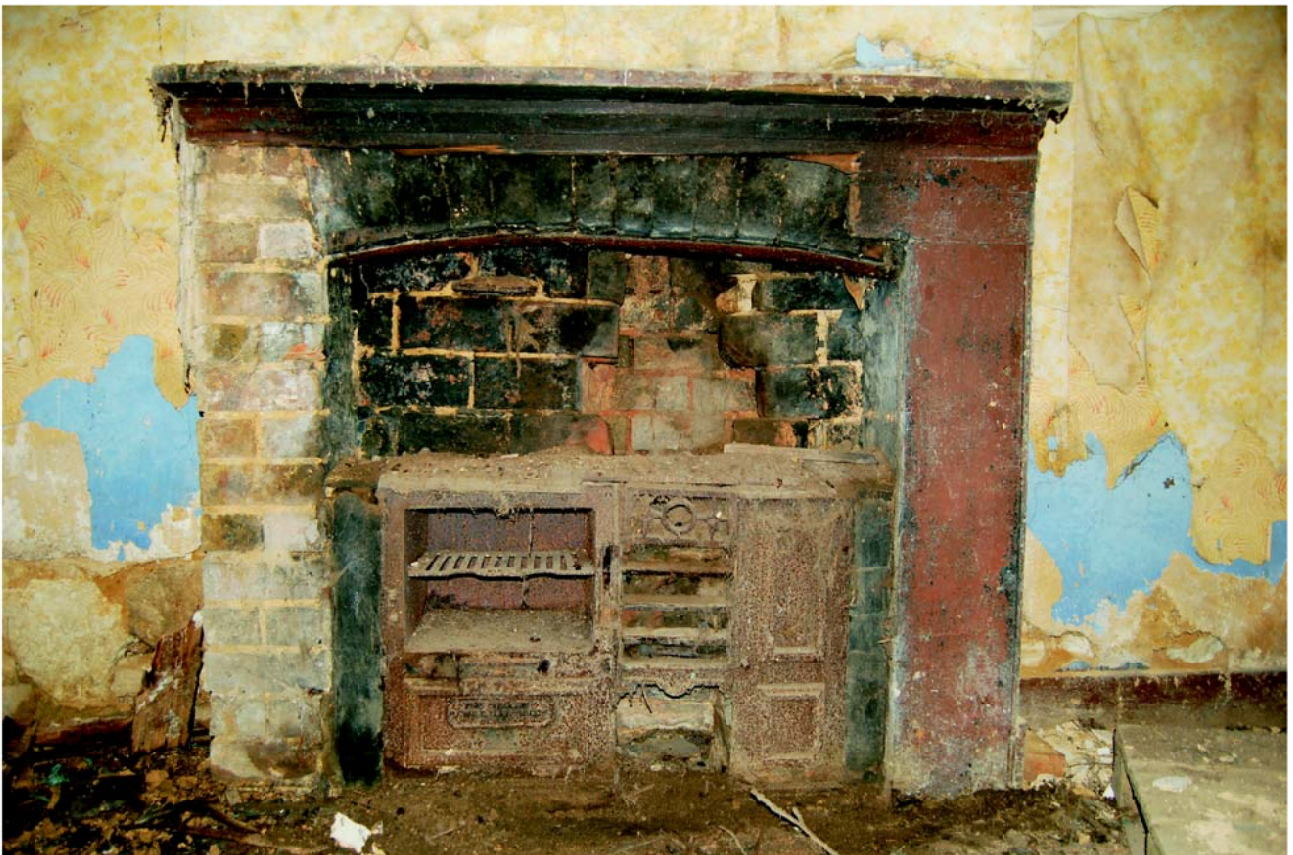
Plate 15: Cast iron stove in Room 3, looking west.
