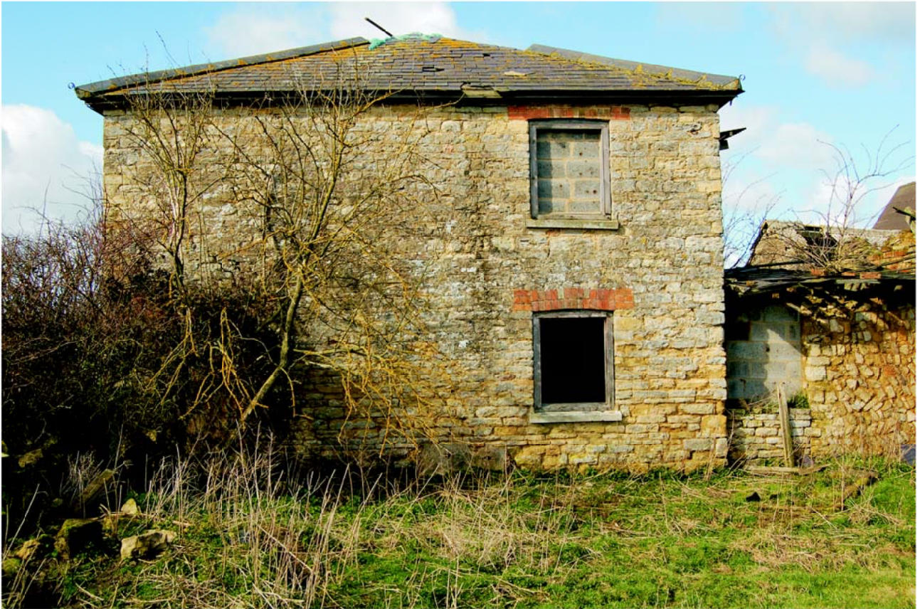
Plate 3: East facade of the farmhouse, looking west
