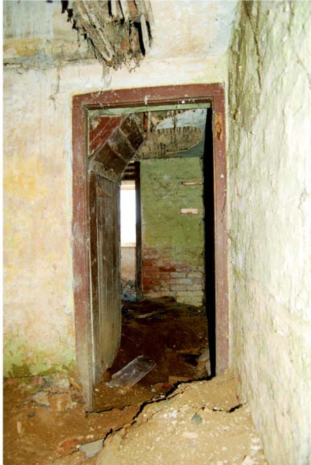
Plate 11: Inserted door between Rooms 1 and 2, looking east.
