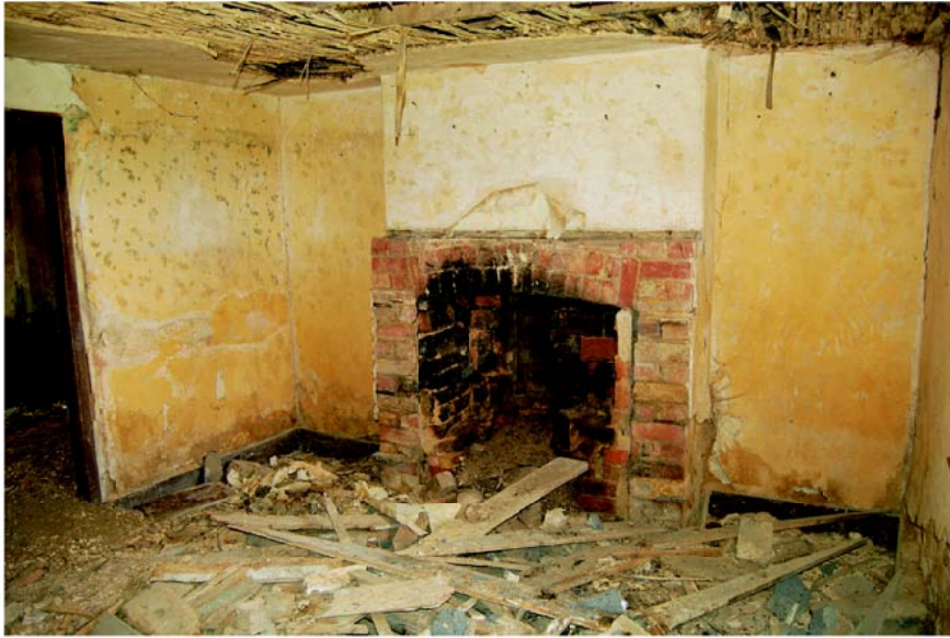
Plate 16: Room 4, looking north-east.
