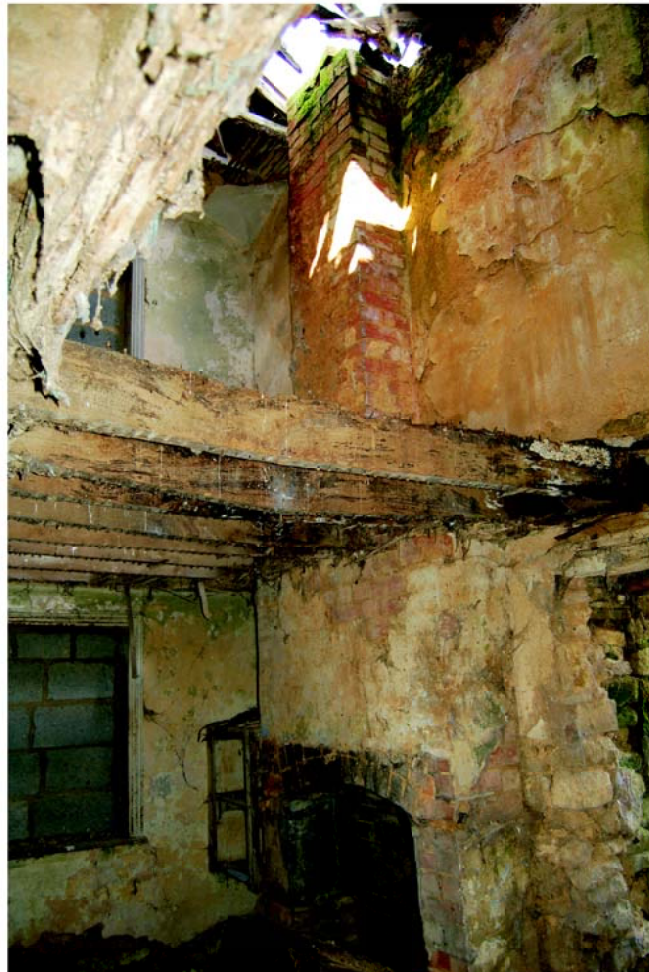
Plate 20: Room 8, looking north-west.
