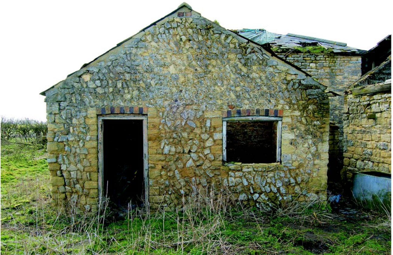
Plate 24: North gable end of Rooms 11 and 12.
