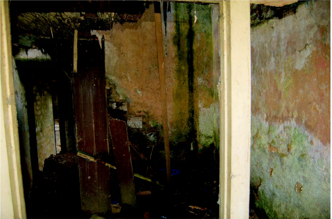
Plate 9: Stairs in Room 2, looking west.
