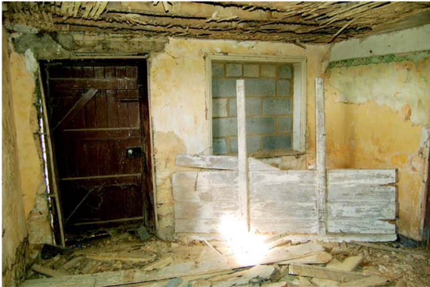
Plate 17: Room 4, looking west.
