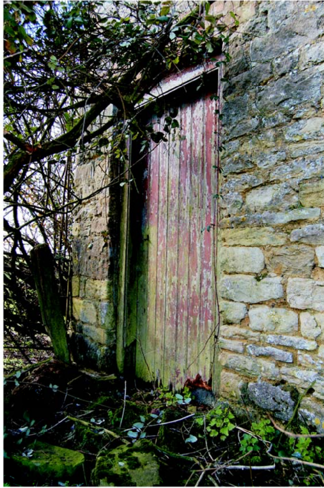
Plate 14: Room 3 door in east wall from outside.
