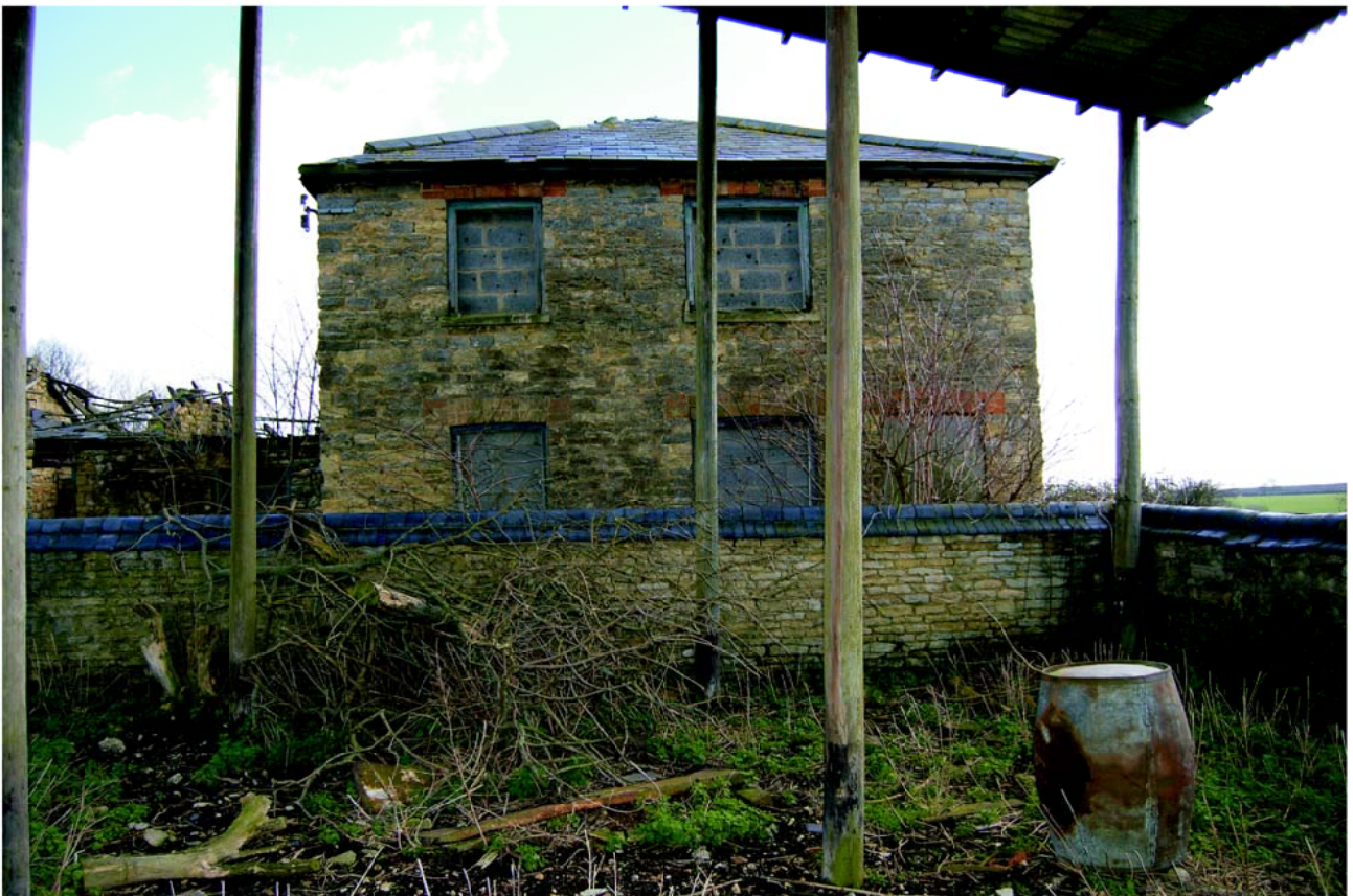
Plate 2: West facade of the farmhouse, looking east.
