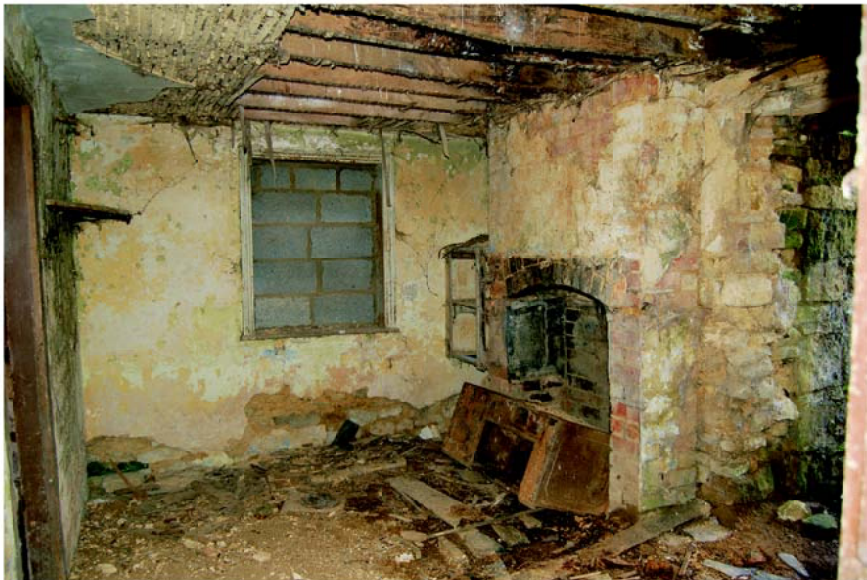
Plate 6: Room 1, looking north-west.
