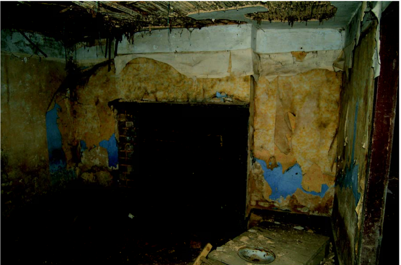
Plate 13: Room 3, looking south-west.
