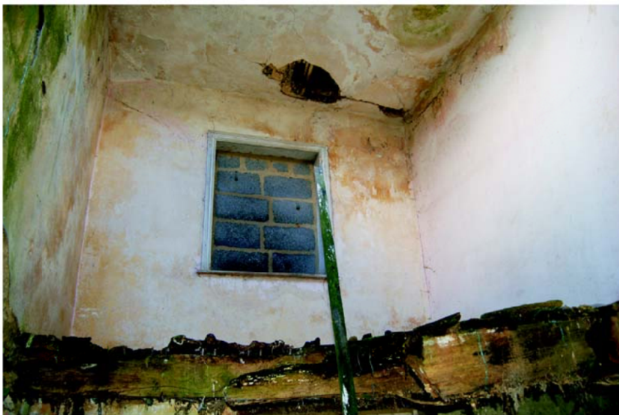
Plate 18: Room 5, looking east.
