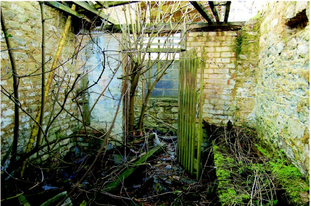
Plate 22: Room 10 slatted door in west wall.
