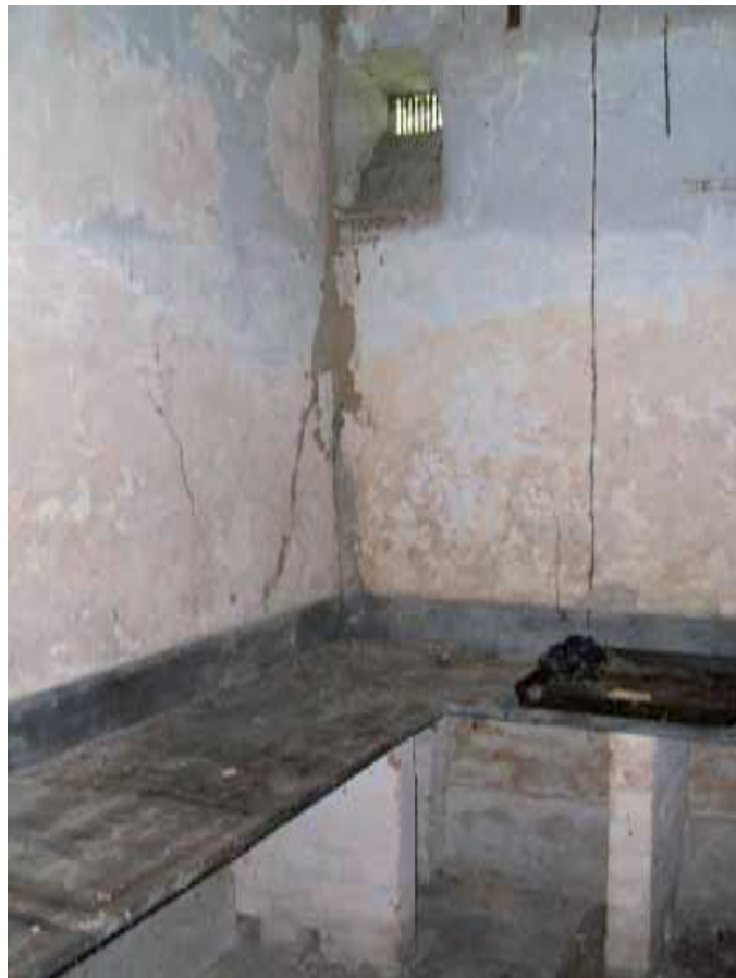
Plate 30: North annexe, slate benches in former larder (N3)
