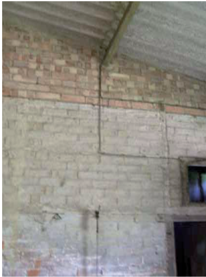
Plate 29: North annexe, brick lift to add current roof to reduced cottage (N2/3).
