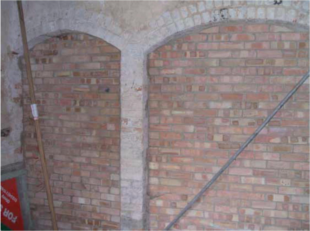
Plate 27: North annexe, blocked arcade in north wall (N1).
