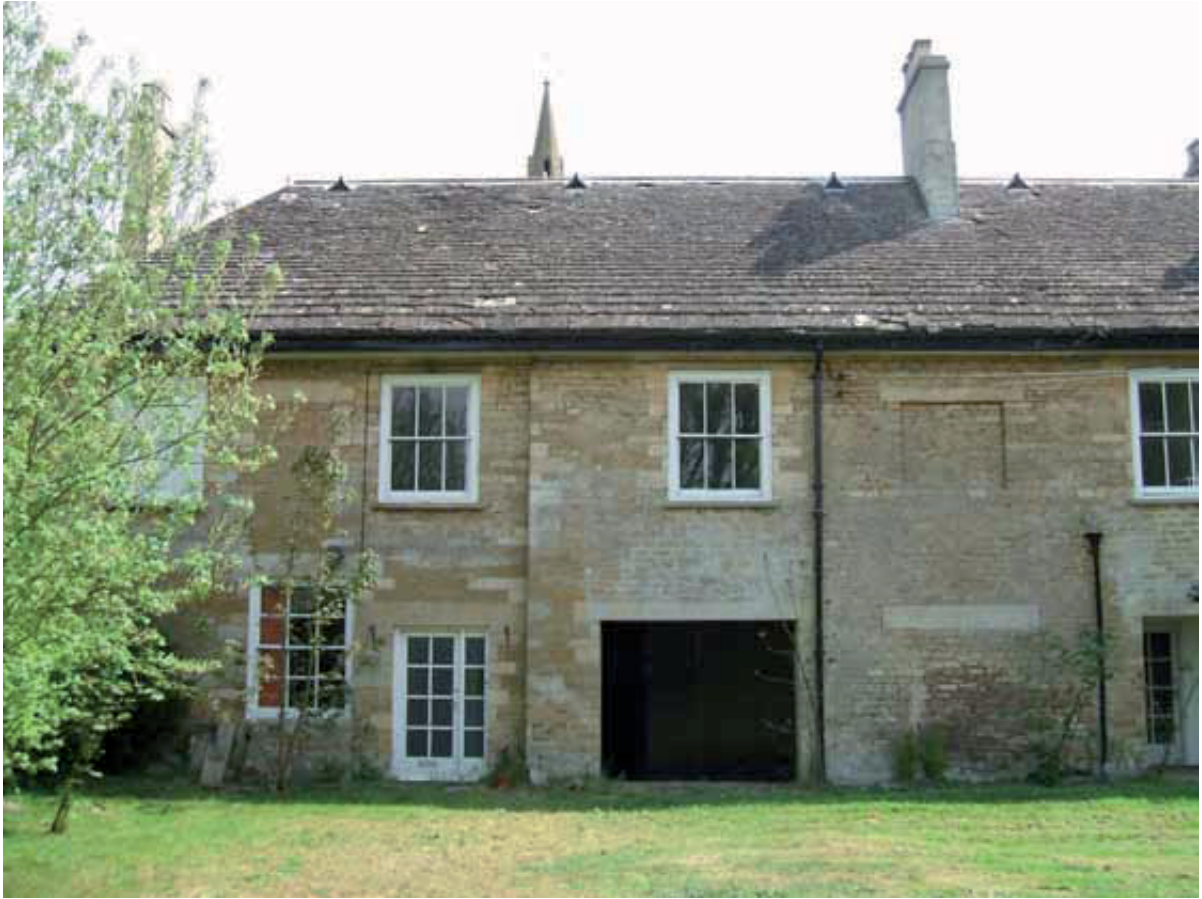
Plate 7: The west, service façade.
