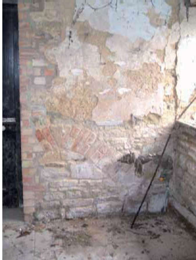
Plate 26: North annexe, brick arch low in east wall (N1).
