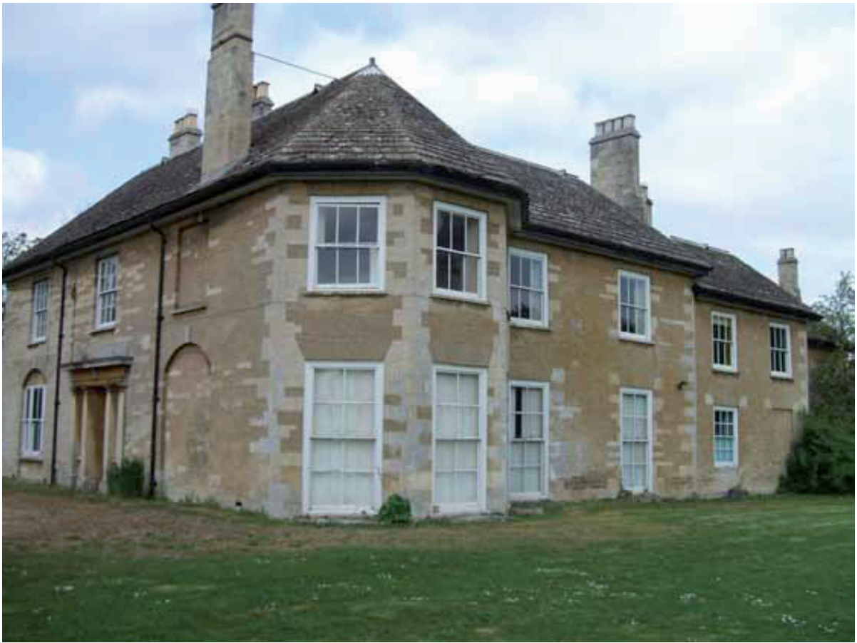
Plate 3: The rectory from the south-east, showing the two main façades.
