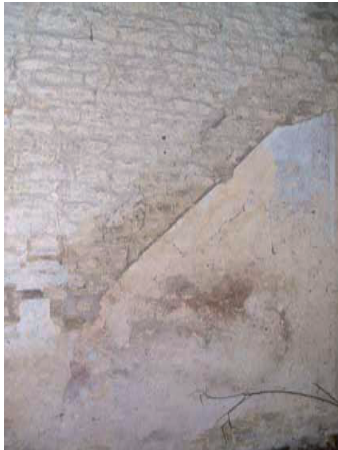
Plate 28: North annexe, scar of former cottage stair (N2).
