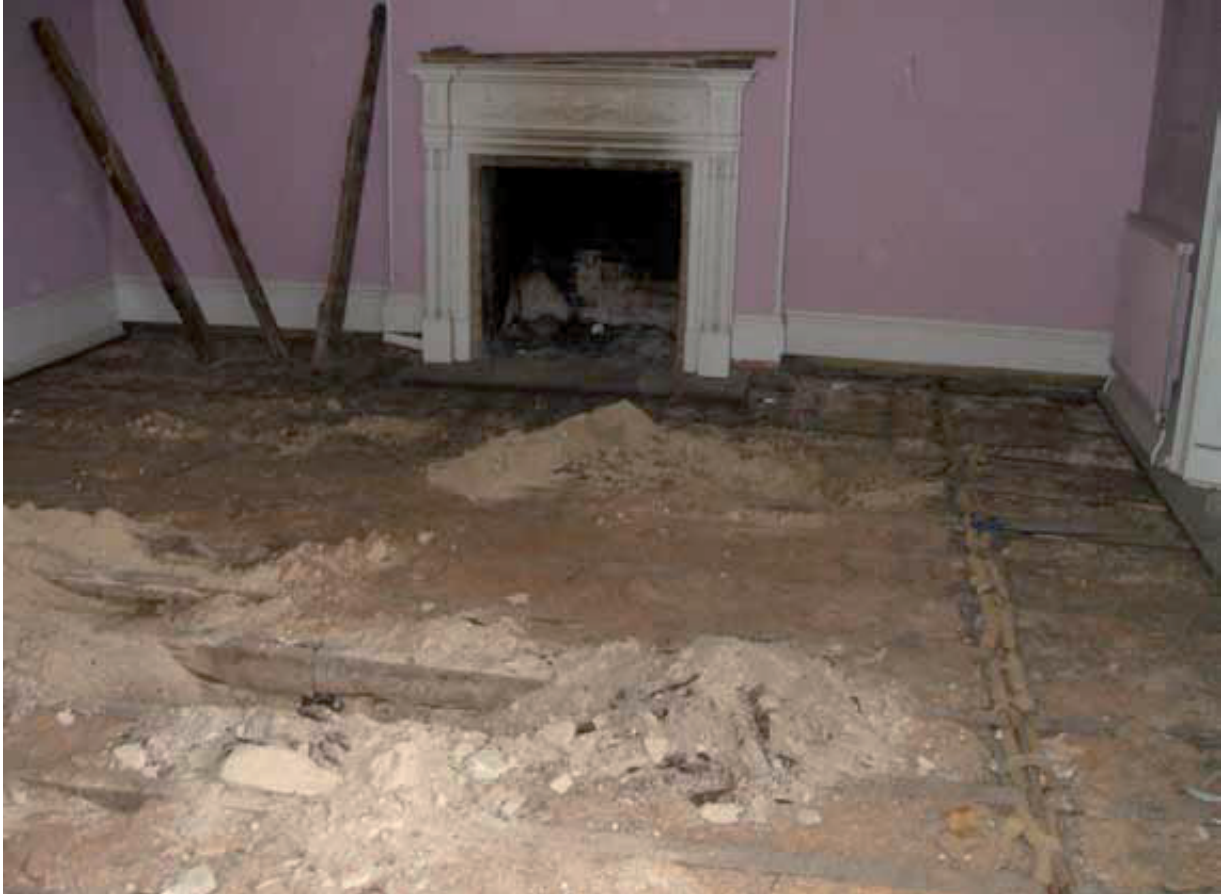
Plate 14: The exposed sub-floor of the dining room.
