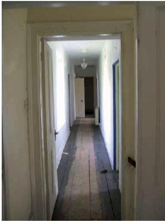
Plate 23: The first floor service corridor.
