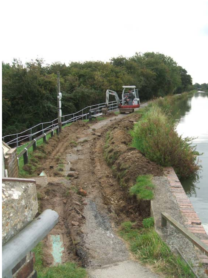
Plate 2: Excavations along edge of towpath. Looking south-east
