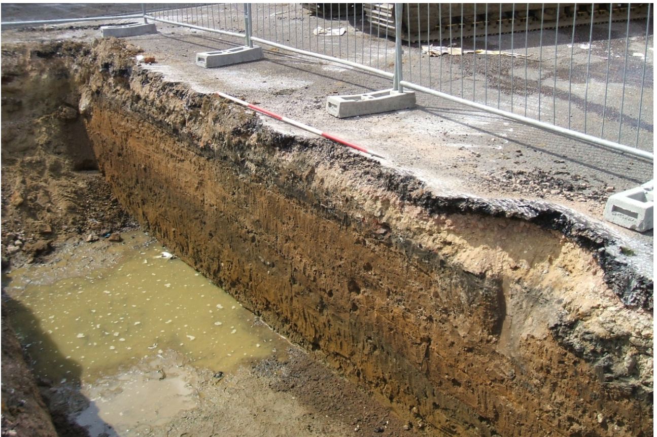
Plate 2: Trench 2, south-west section facing south.
