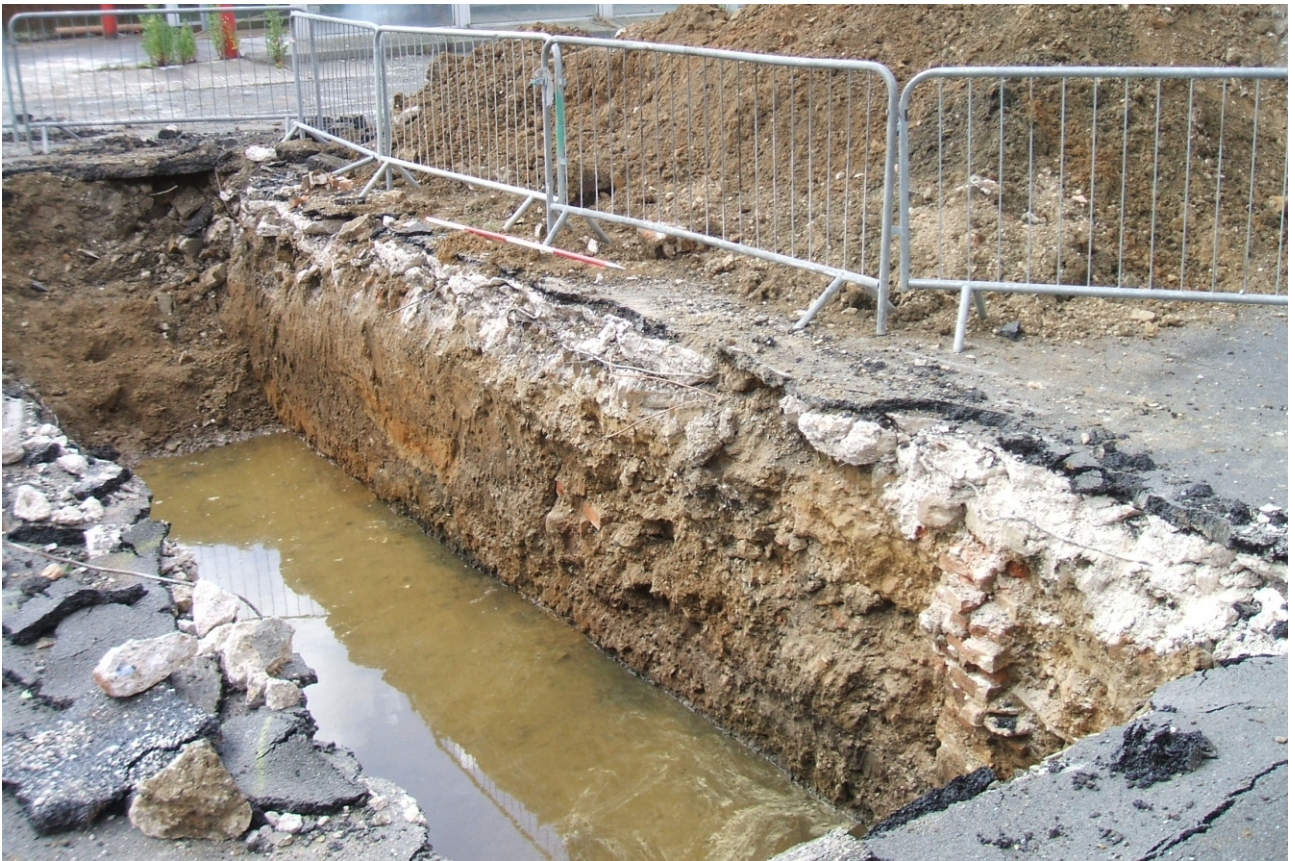
Plate 1: Trench 1, south-west section facing south.
