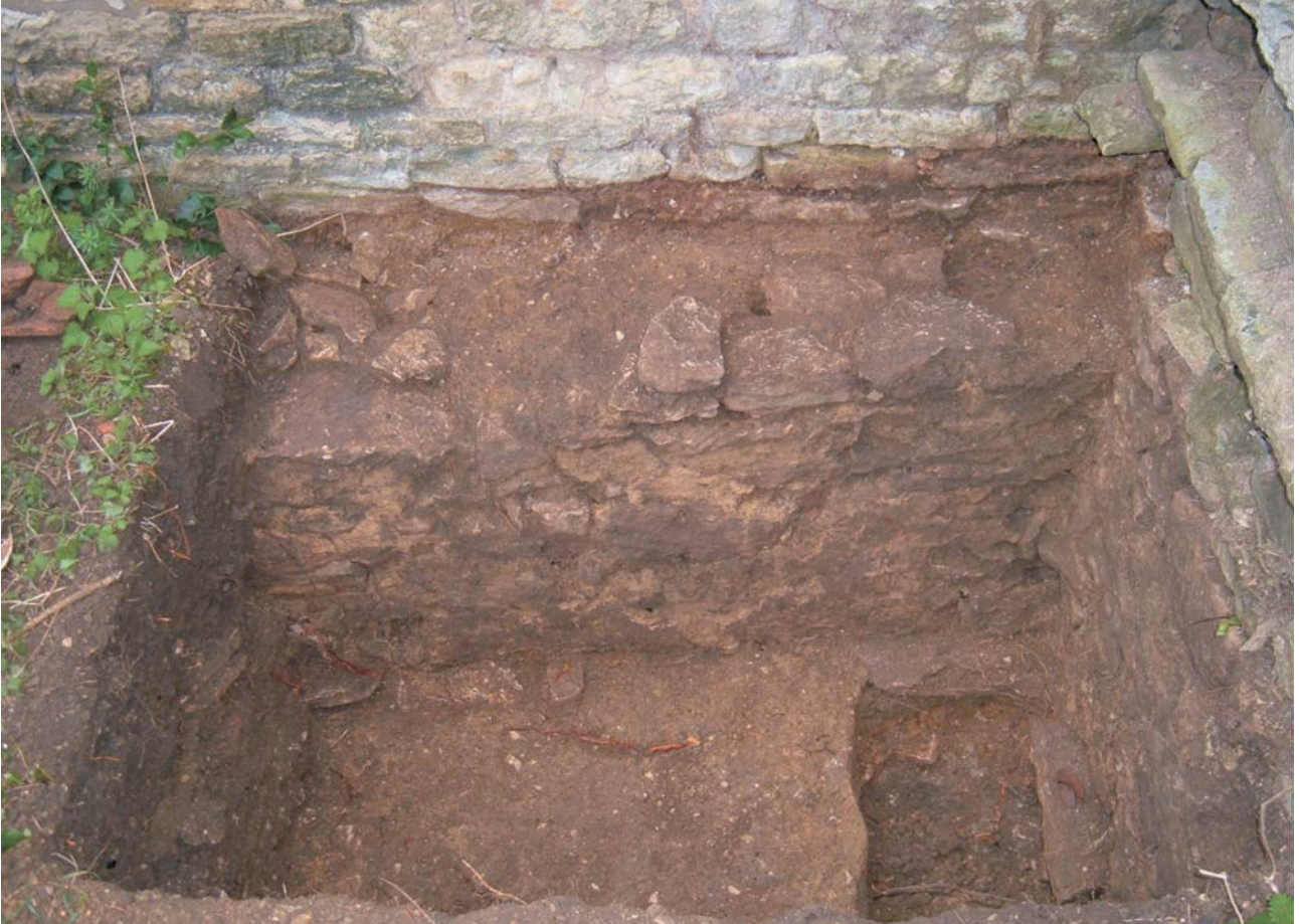
Plate 8: Test Pit 2, floor surface, construction trench and lower wall courses.
