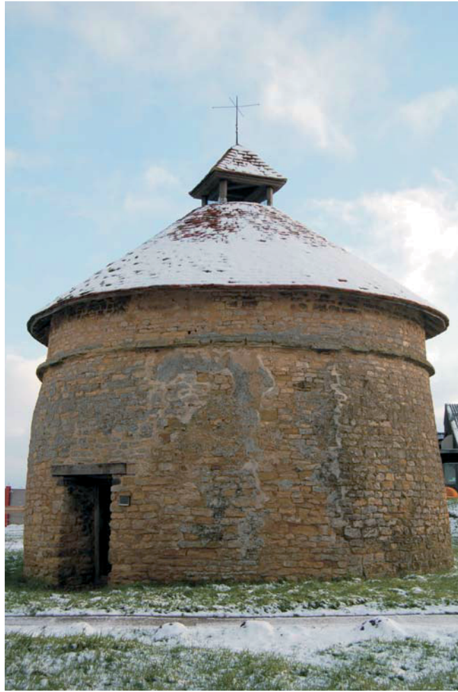
Plate 1: Furtho dovecote c15th century.
