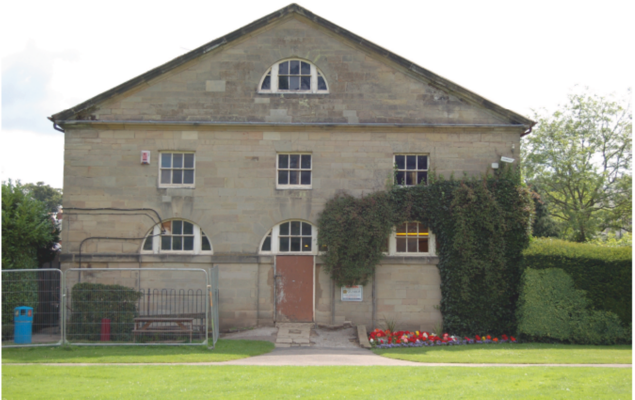
Plate 1: West façade of the building.
