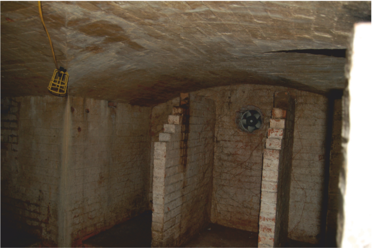
Plate 21: Brick wine-bin divisions in Room 37.
