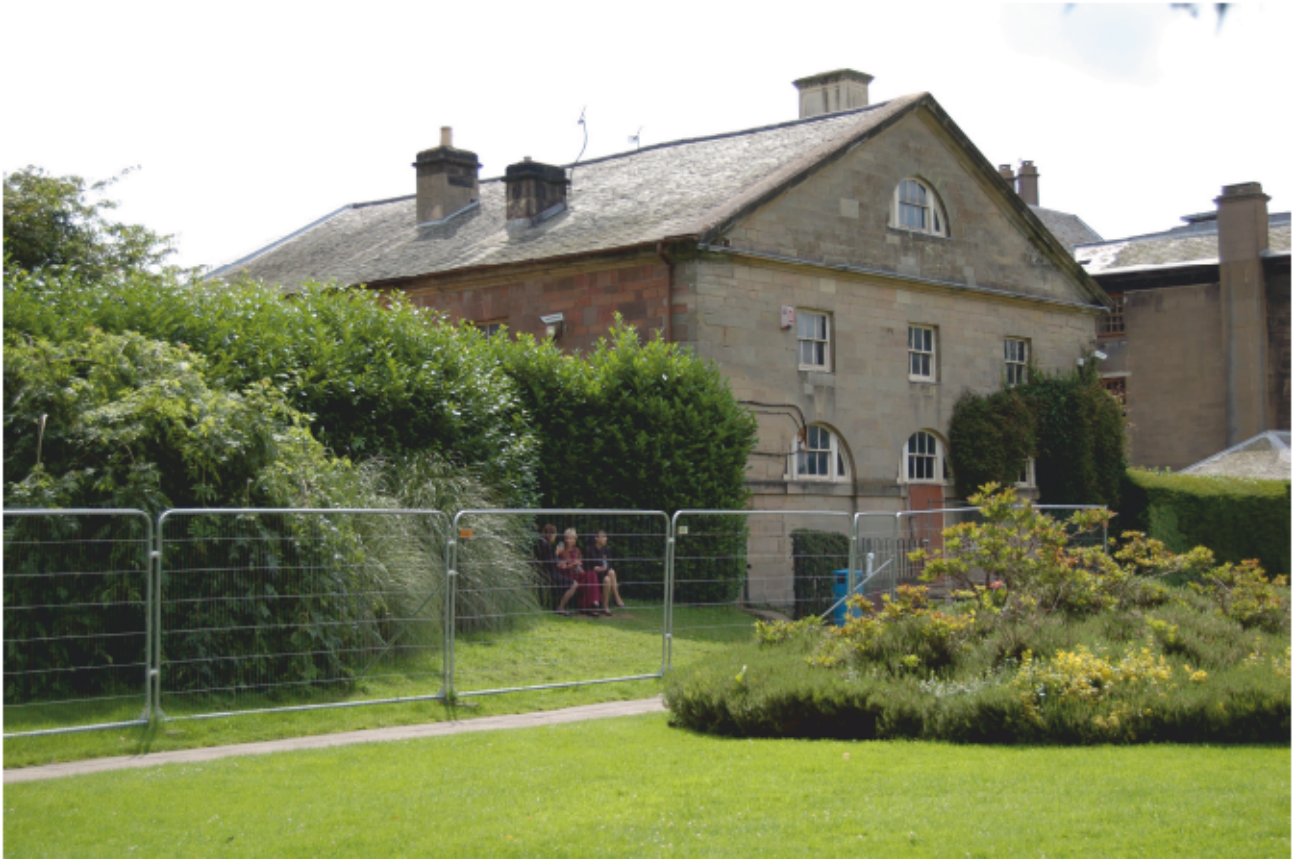
Plate 9: Building looking south-east showing chimneys on north side.
