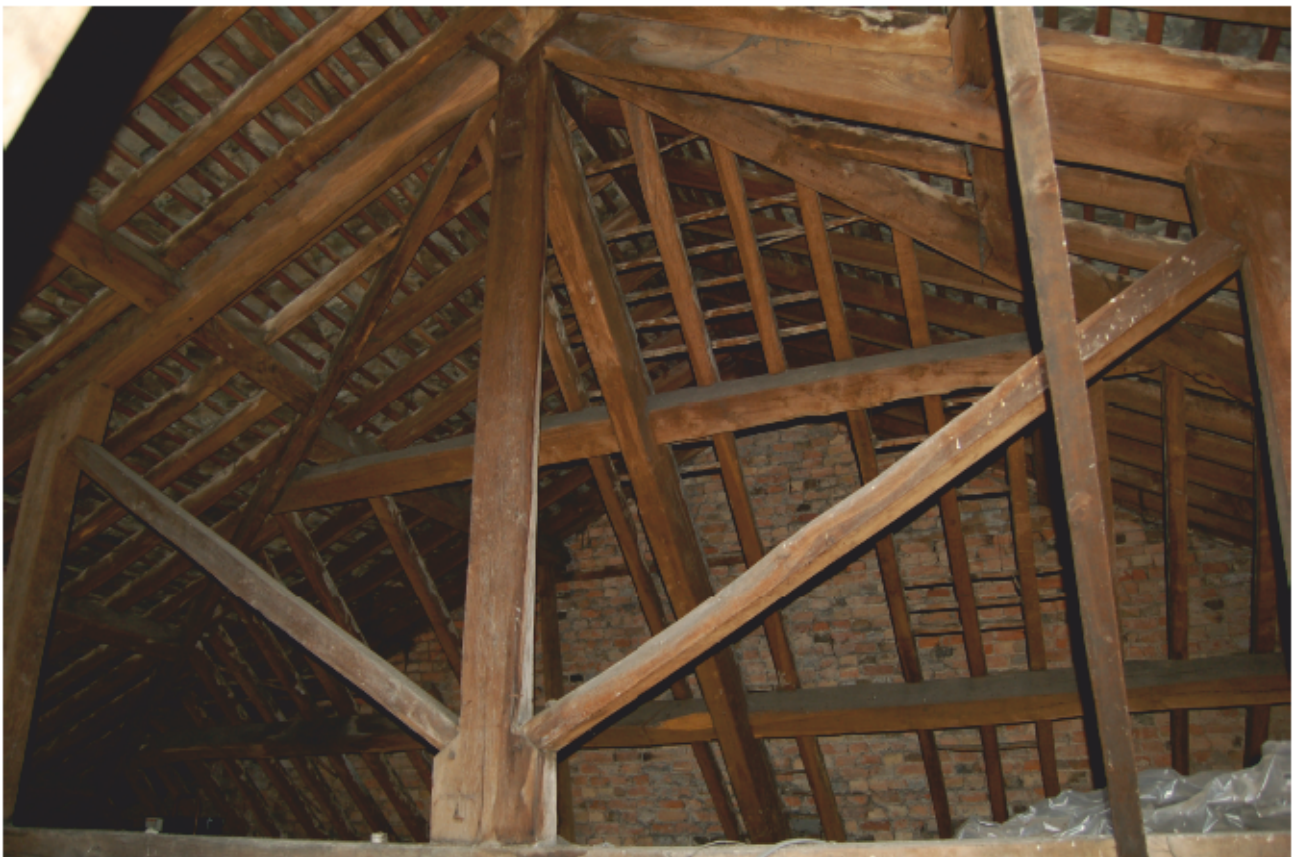
Plate 14: Timbers of original hipped roof looking east.
