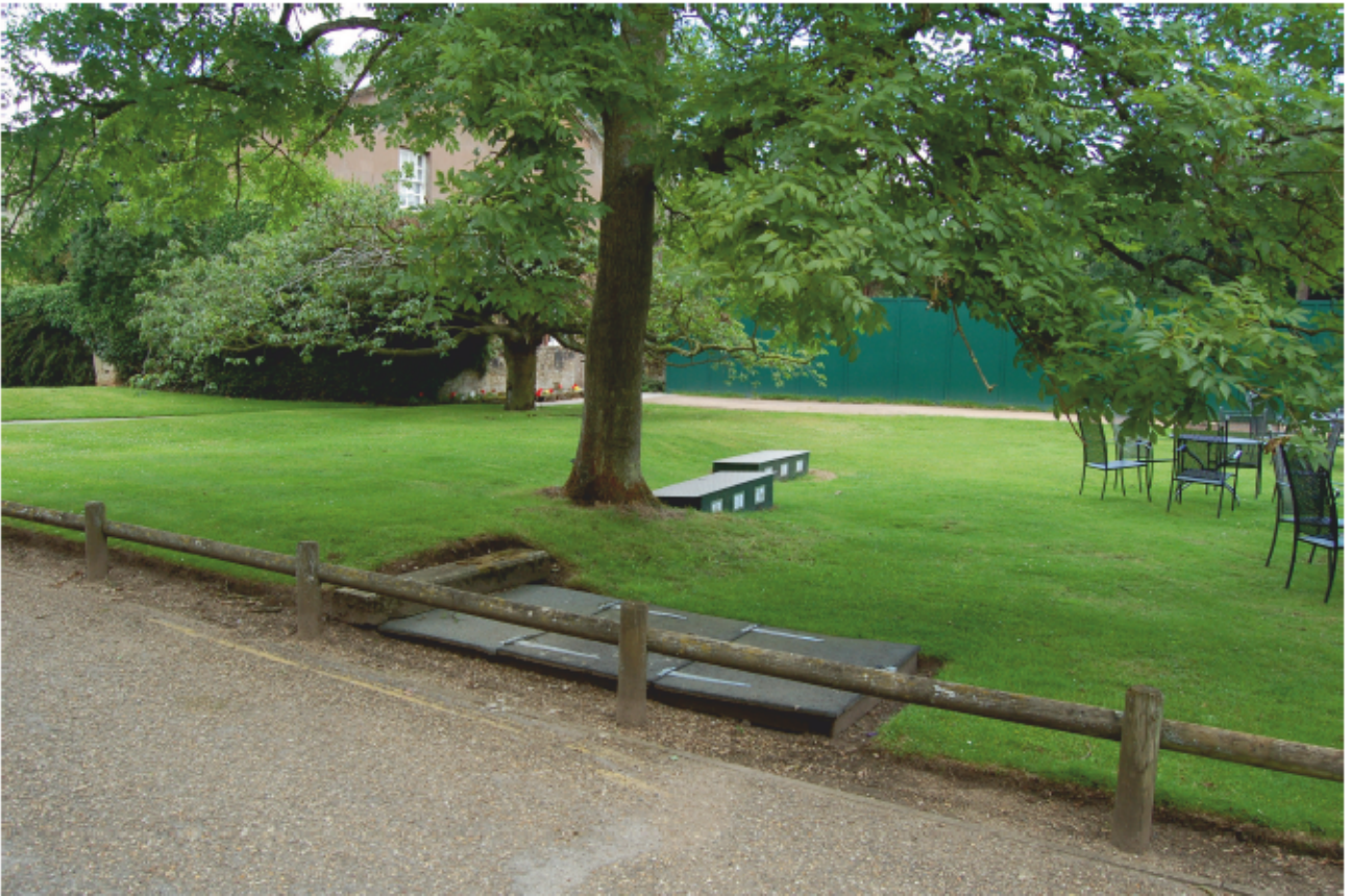
Plate 23: Modern coverings for cellar steps from Room 39 (foreground) and two light-wells (background).
