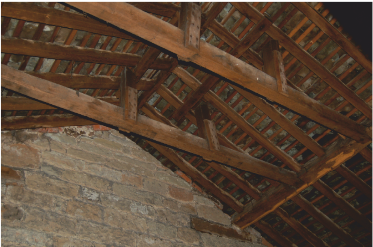
Plate 16: Stubs of possible cupola structure.
