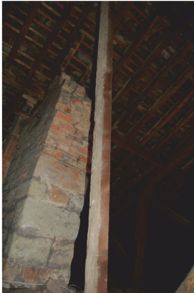
Plate 15: South side of chimney stack, note the stub of brick linking arch.
