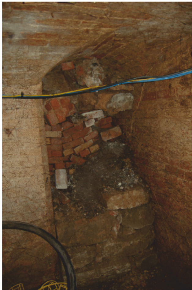
Plate 20: Blocked cellar corridor at east end of Room 34.
