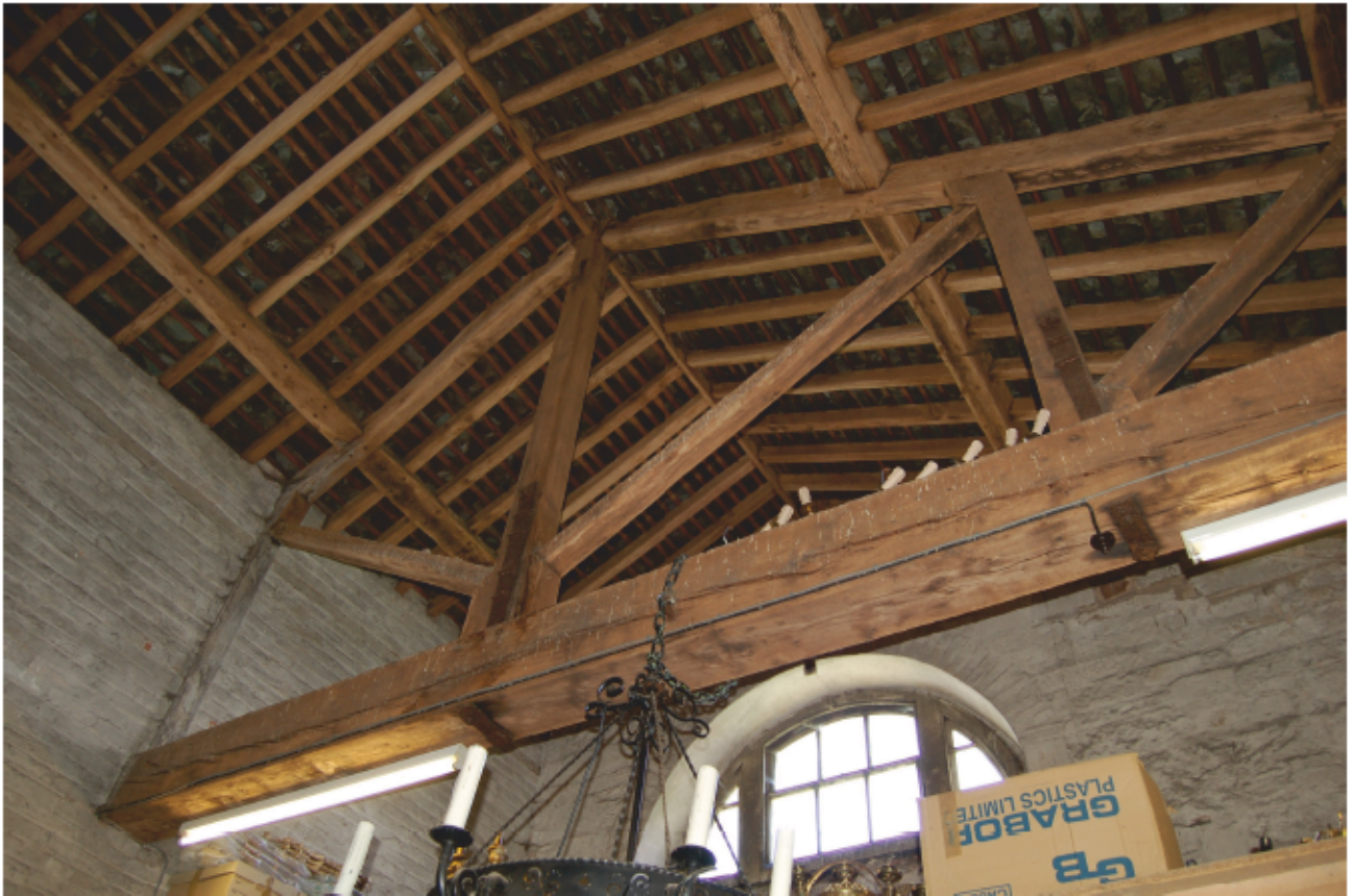
Plate 11: Truss of Room 18.
