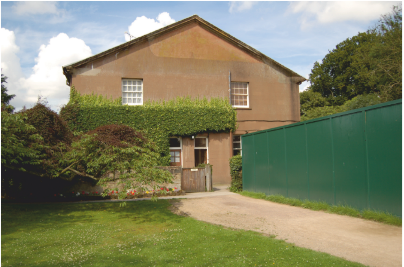
Plate 3: East façade of the building.
