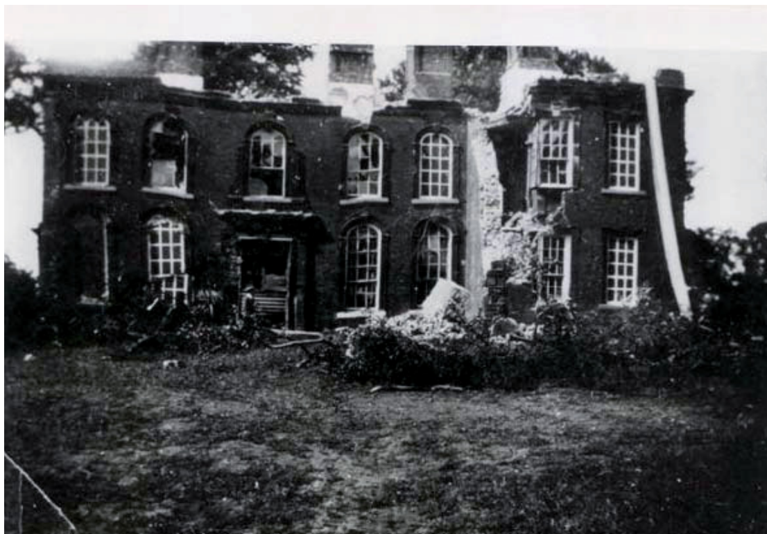
Plate 5: Bentley Hall demolition 1929 (from a photo supplied by Sally Birch)
