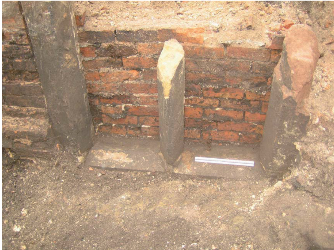
Plate 15: Trench 8 – window (807) detail
