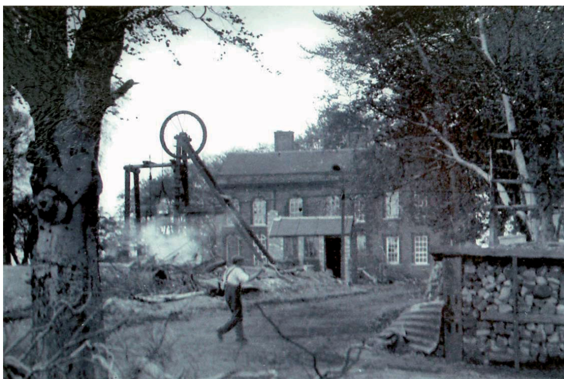
Plate 4: Bentley Hall with mine winding gear circa 1926
