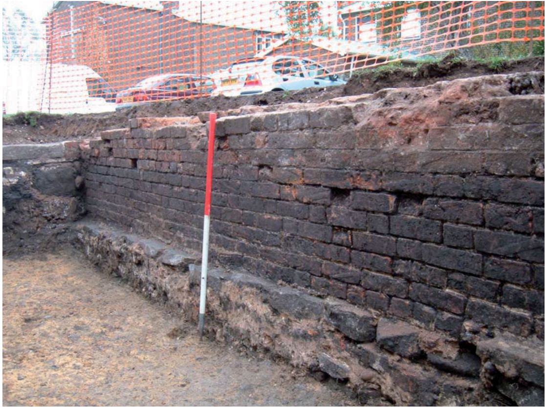
Plate13: Trench 8 – wall (803) on foundation (805)
