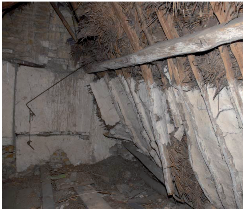
Plate 4: The attic interior showing the whitewashed plastered thatch
