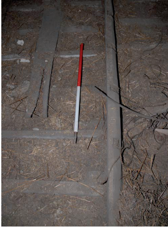
Plate 5: The attic floor
