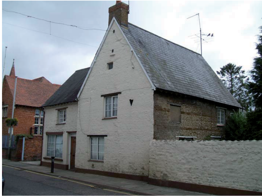
Plate 1: The exterior showing the ironstone banding on the southern elevation
