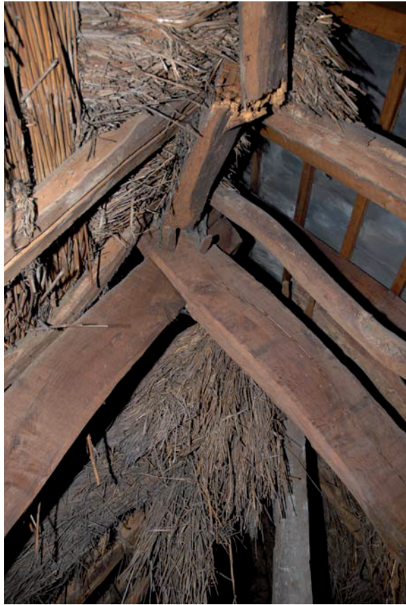
Plate 3: Joint detail of the principal rafter
