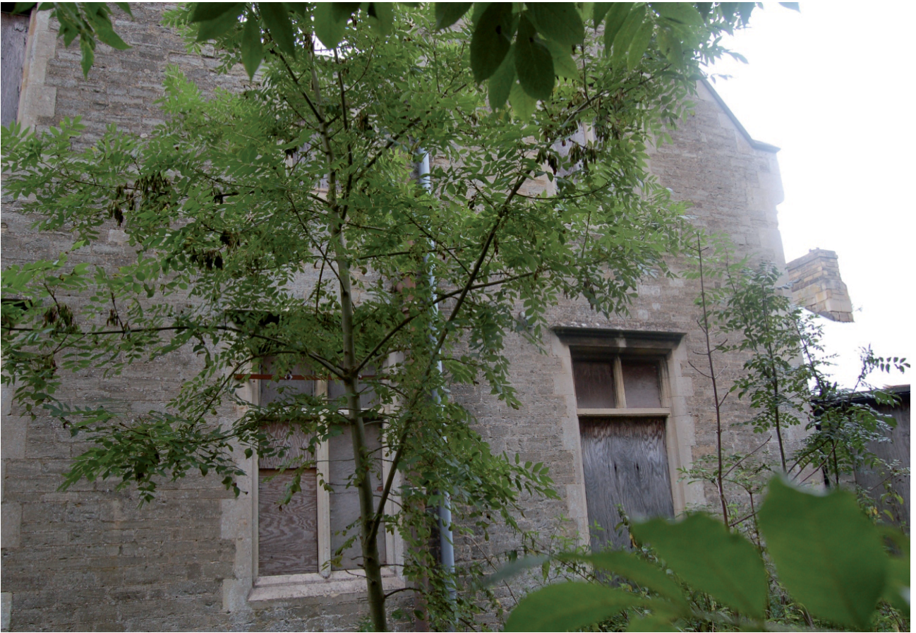
Plate 5: West facade looking east
