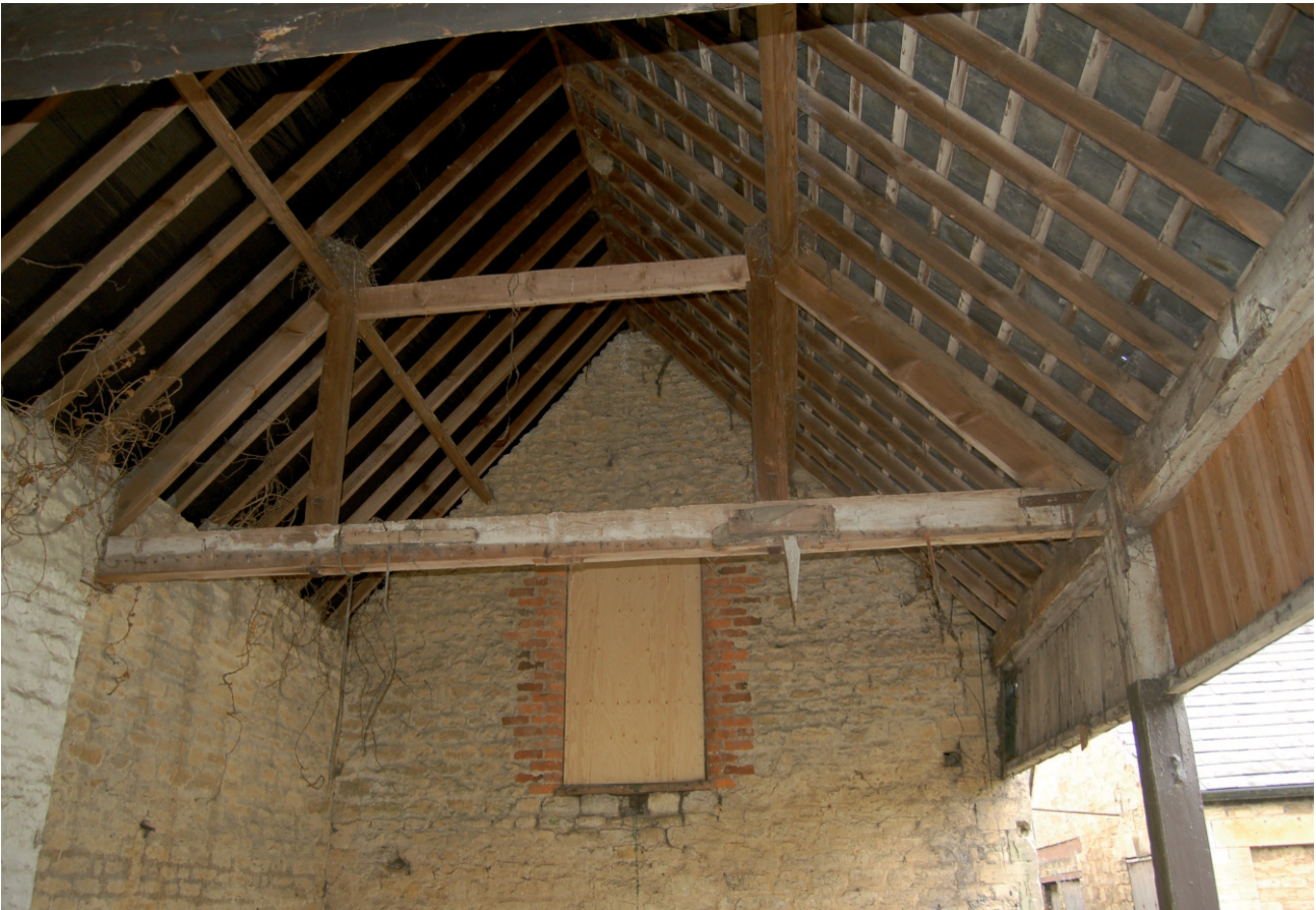
Plate 8 Roof structure of barn looking west showing roof truss and hayloft door from two-storey western section
