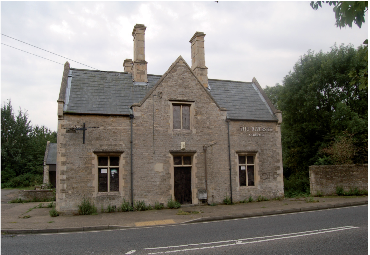
Plate 3 North facade looking south
