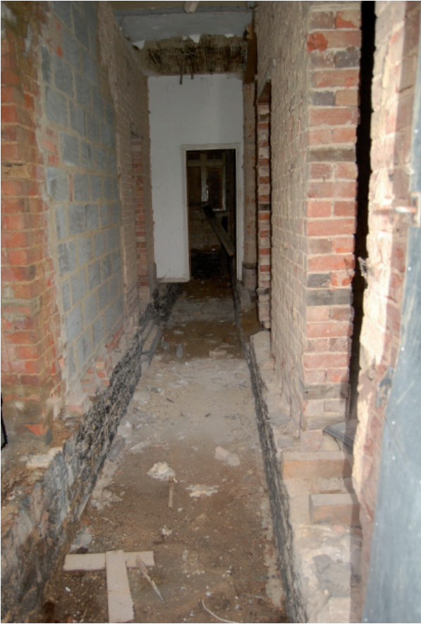
Plate 9 Central corridor of hotel looking west from door in east facade
