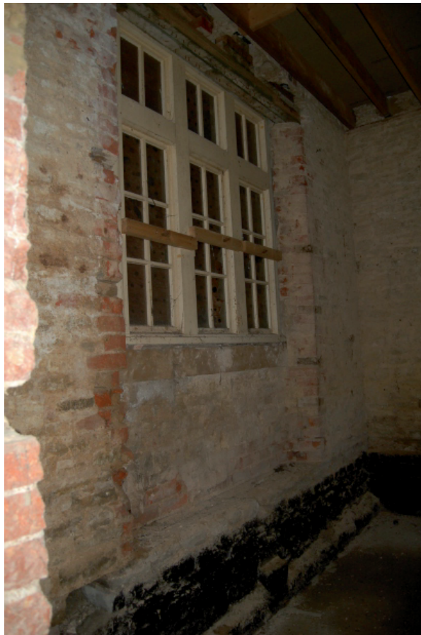
Plate 2 Window of room on east front showing window frame
