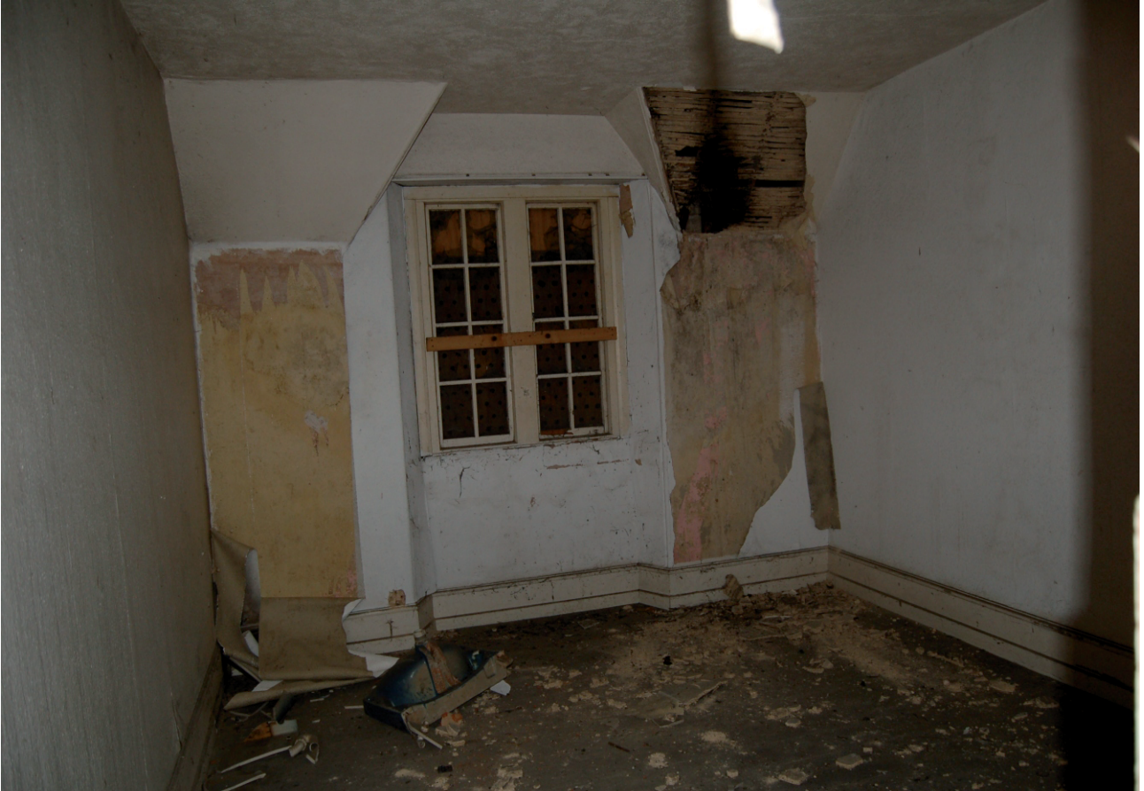
Plate 11 Bedroom on south side of building with cross-eaves window looking south
