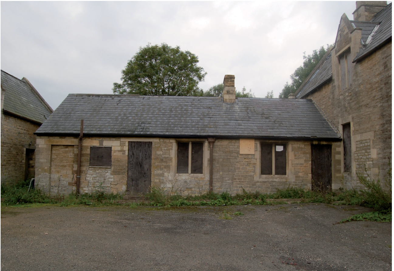
Plate 6: East side of single storey range looking west
