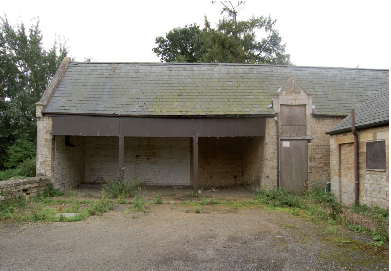
Plate 7 Barn looking south - cart hovel eastern end and hayloft door to first floor towards western end
