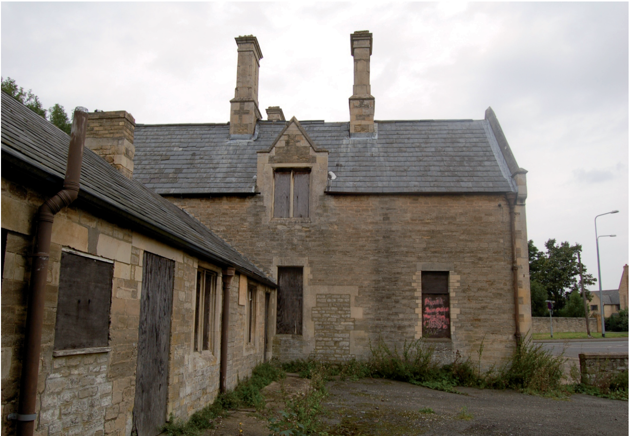
Plate 4 South facade looking north
