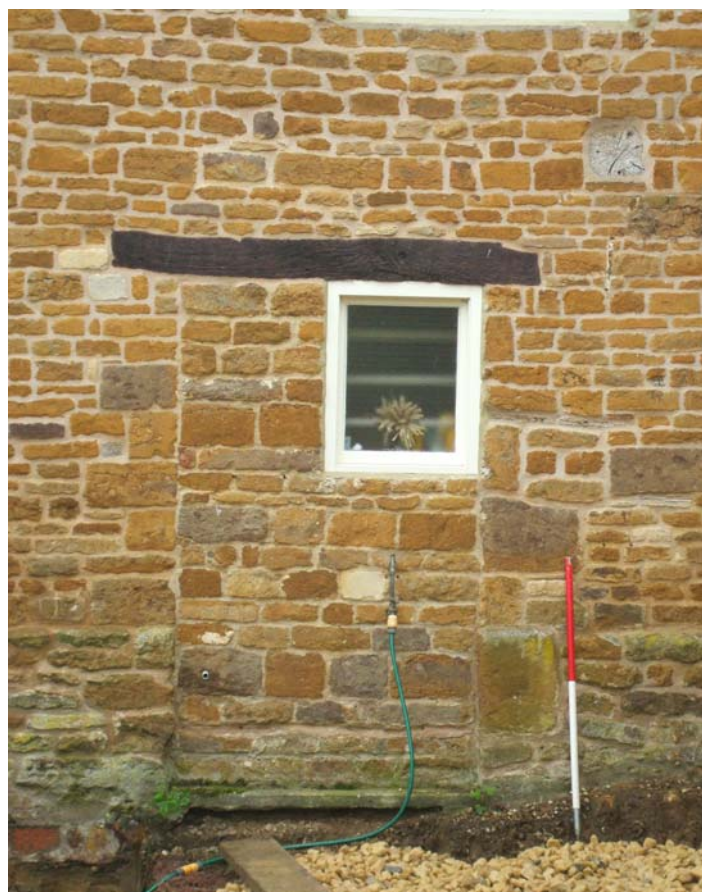
Plate 3: Blocked doorway in the north-west elevation, is set beneath an oak lintel and has a small fixed modern window set within the former opening.
