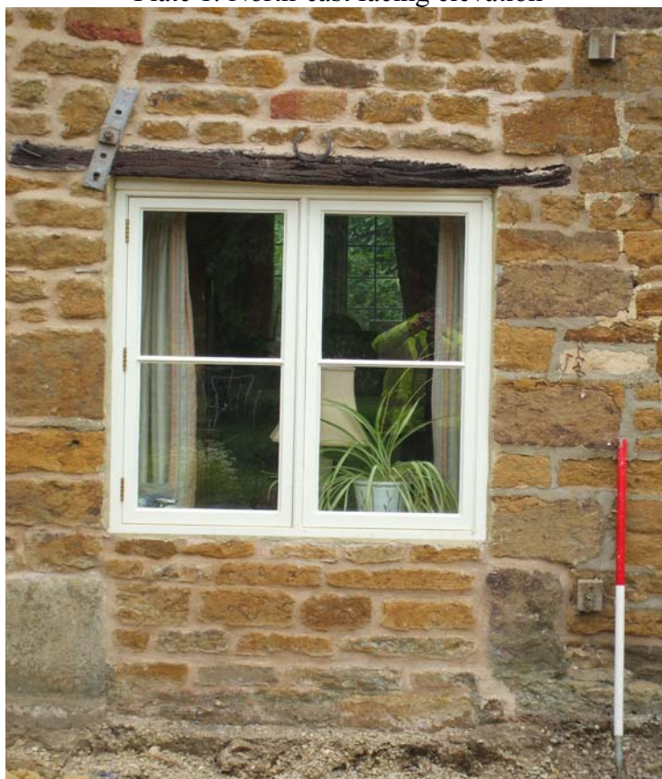
Plate 2: Former doorway in the north-east facing elevation, now half blocked and fitted with a modern casement window beneath the original oak lintel with a modern iron tie set just above it
