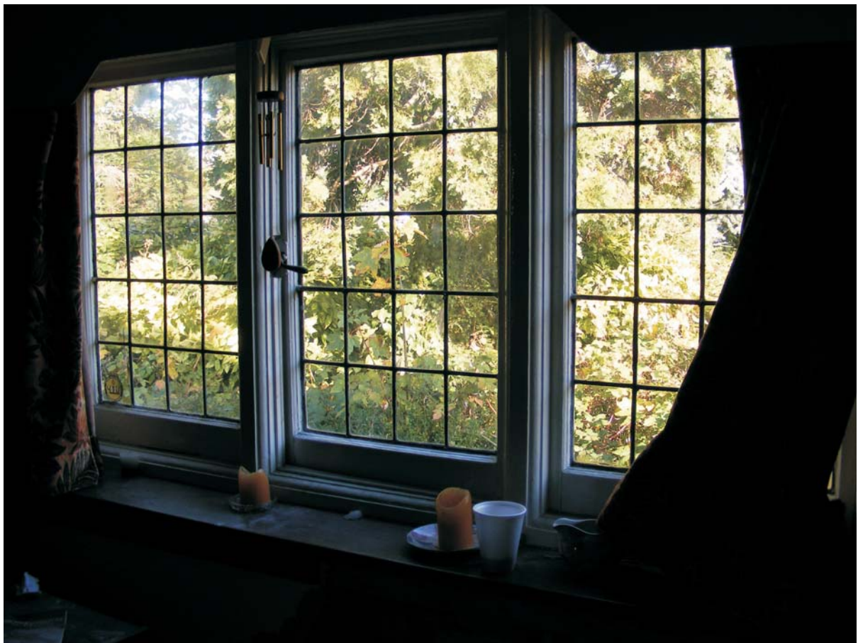
Plate 4: Front room: east facing, leaded casement window
