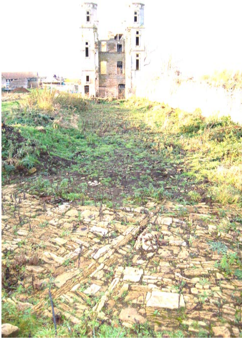
Plate 5: The pitched-stone surface in the South Court, looking north.
