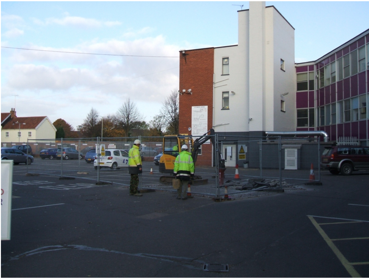
Plate 1: Breaking out Trench 19 in the car park area, looking north-west.
