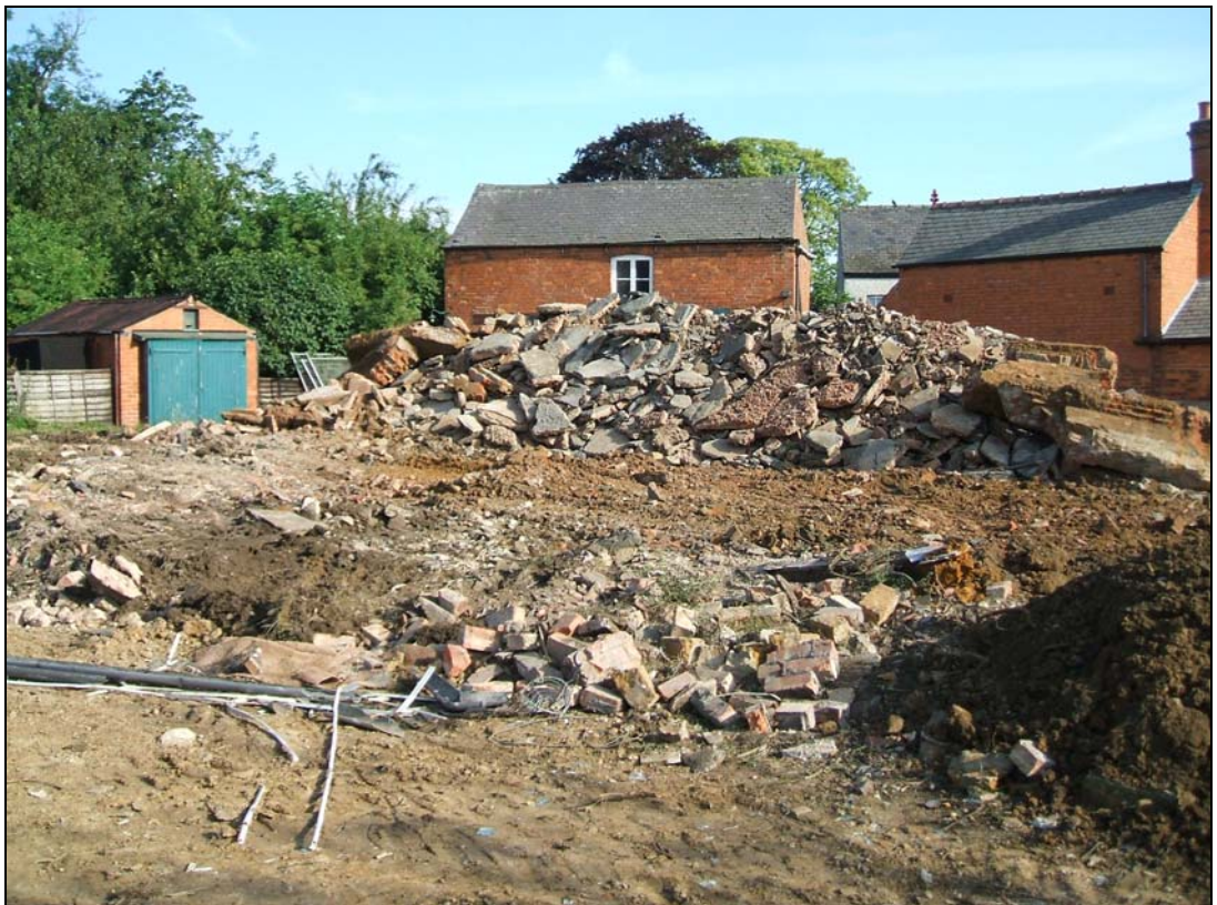
Plate 2: Northern area of site after the demolition of the old farmhouse
