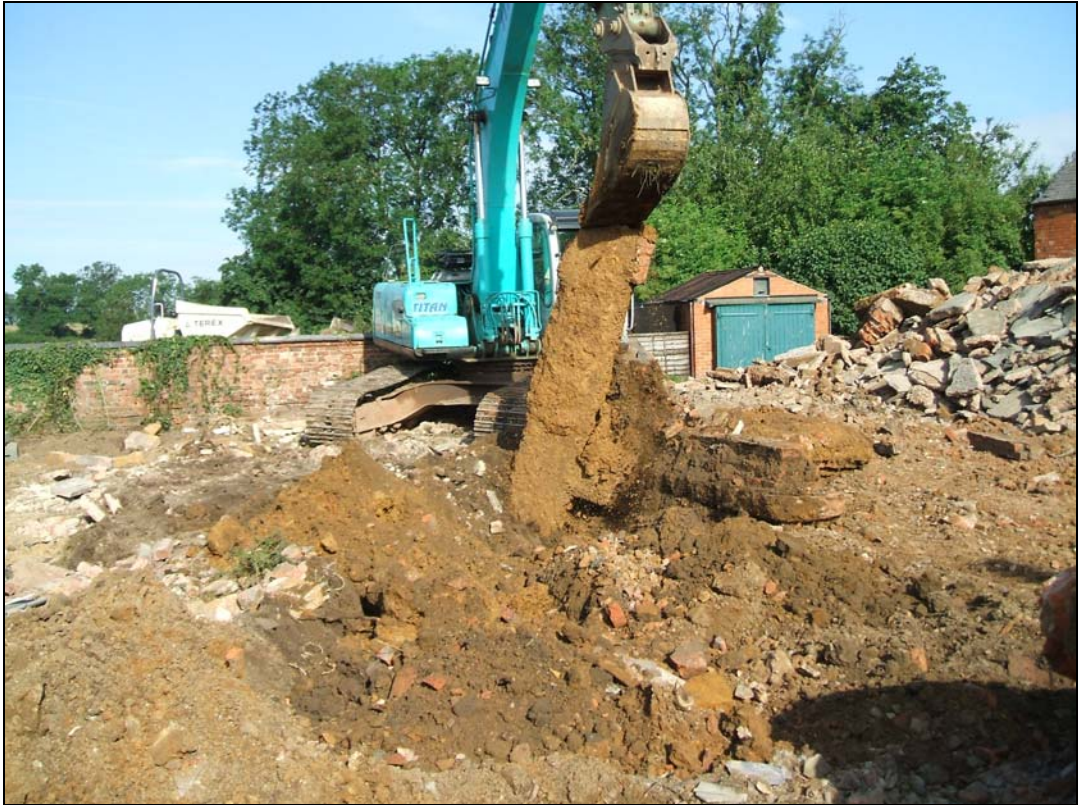
Plate 3: Machine excavating the foundations of the old farmhouse
