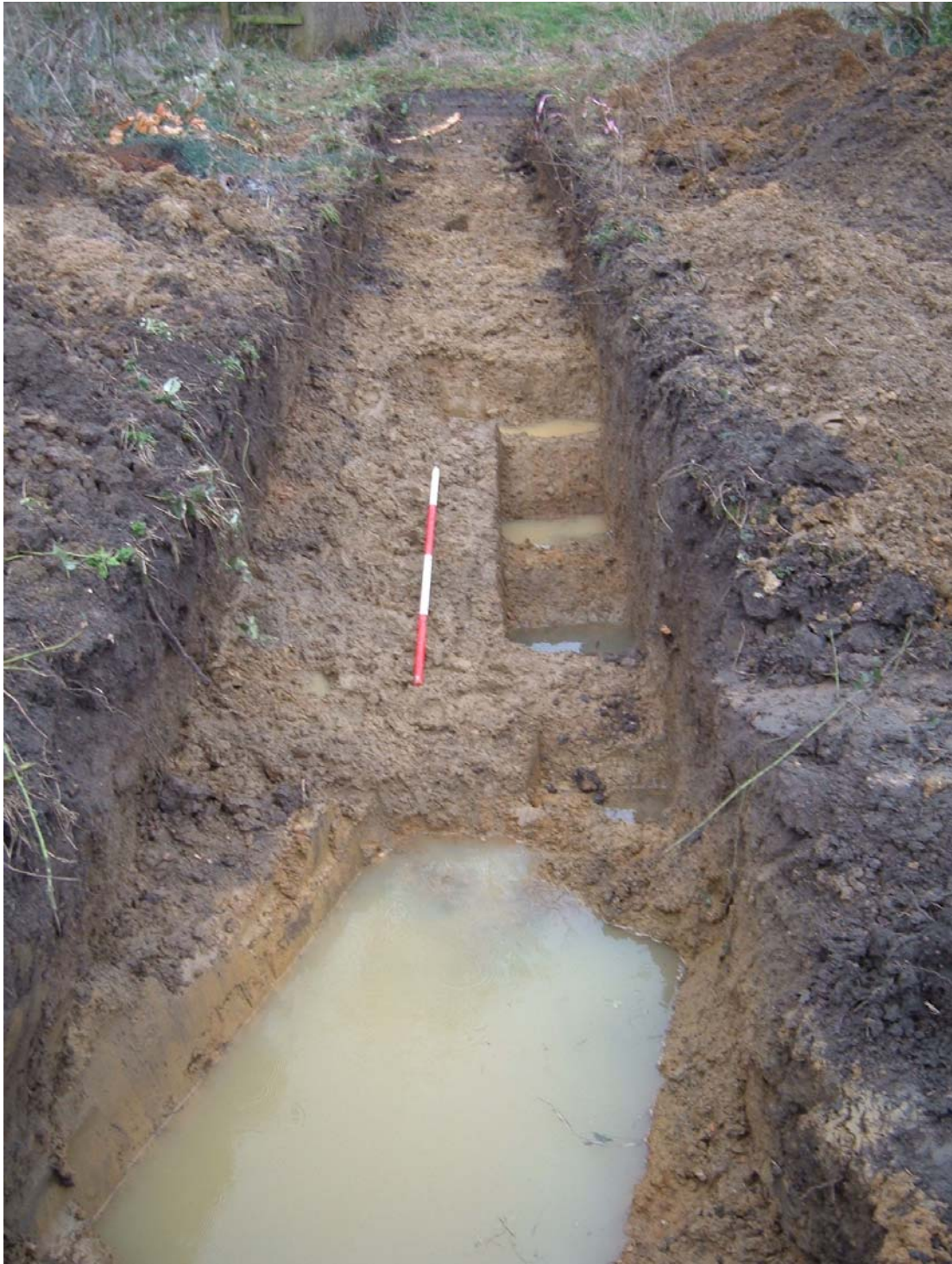
Plate 1: Trench 4, showing ditches [402], [404], [407], [409] and [411], looking west
