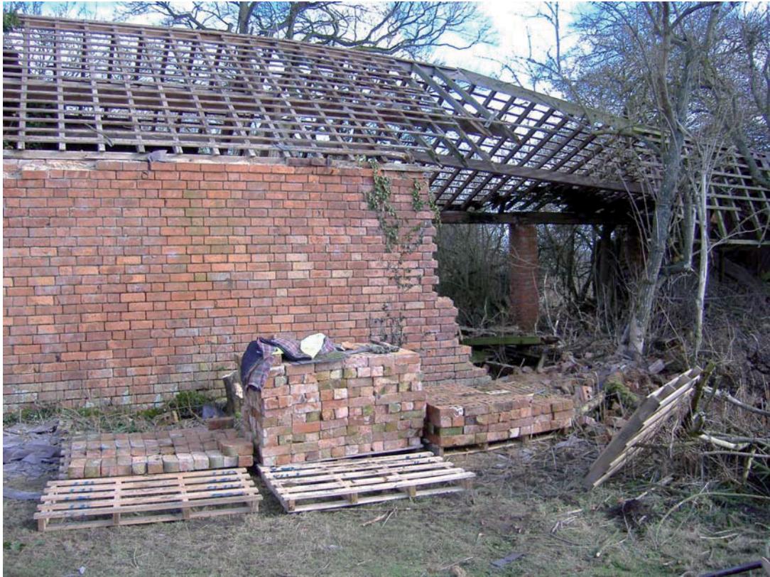
Plate 1: The derelict buildings during demolition, view towards the east
