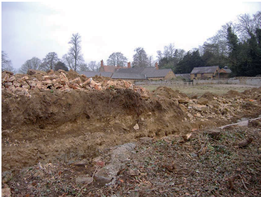
Plate 3: The wall trench in the area of the derelict buildings
