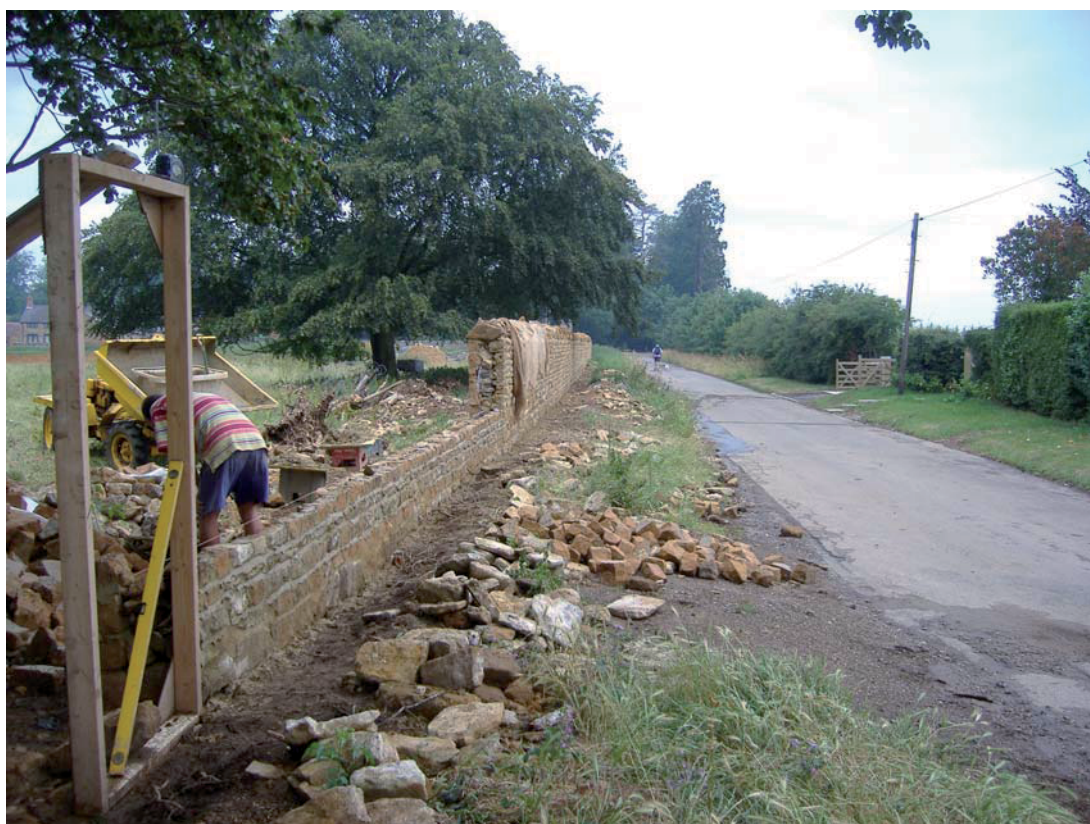
Plate 4: The new wall during construction, viewed to the north
